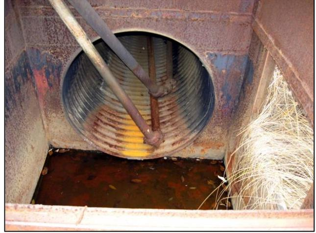
Figure 09 Decant Weir Discharge Culvert Inlet
