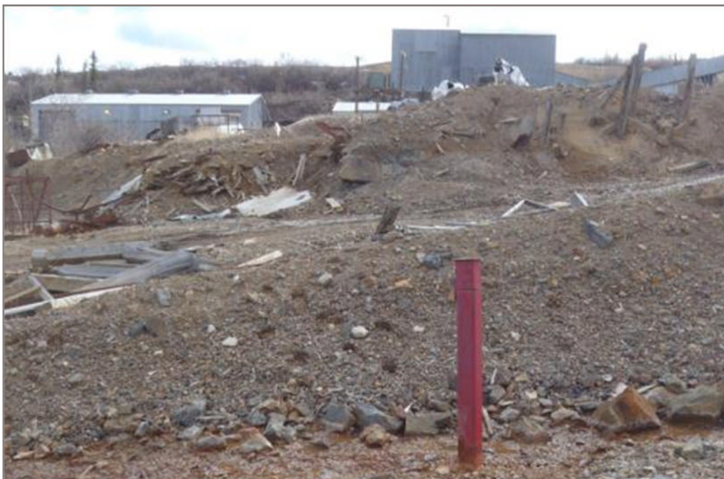
Photo 8: MW09-16 Northeast and Downgradient of the Mill Complex. Note the main mill building in the background. June 1, 2012
