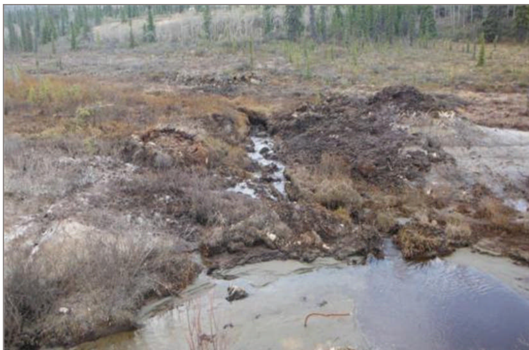
Photo 27: MP09-13 Located in the Dome Creek Diversion at the Intersection of Dome Creek. Note that this Drive-point well is destroyed. June 4, 2012
