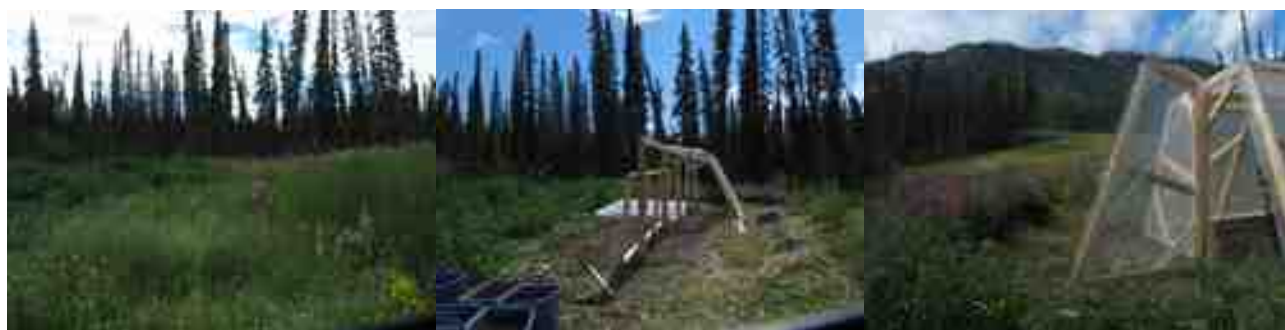
Figure 2 – McClintock Valley site, shelter under construction, and completed
