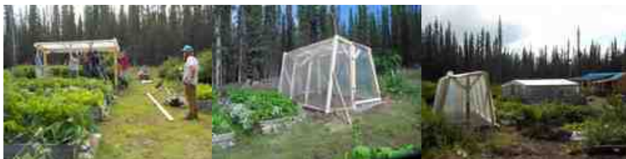
Figure 4 – Annie Lake shelter under construction and complete
