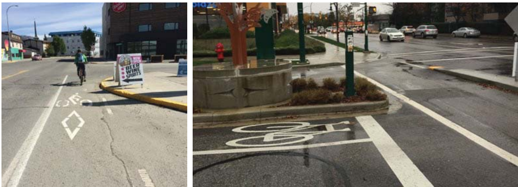
[Left] City of Whitehorse – Bicycle Lane Un-Buffered [Right] City of Vancouver – Bicycle Lane with Bicycle Push Button
