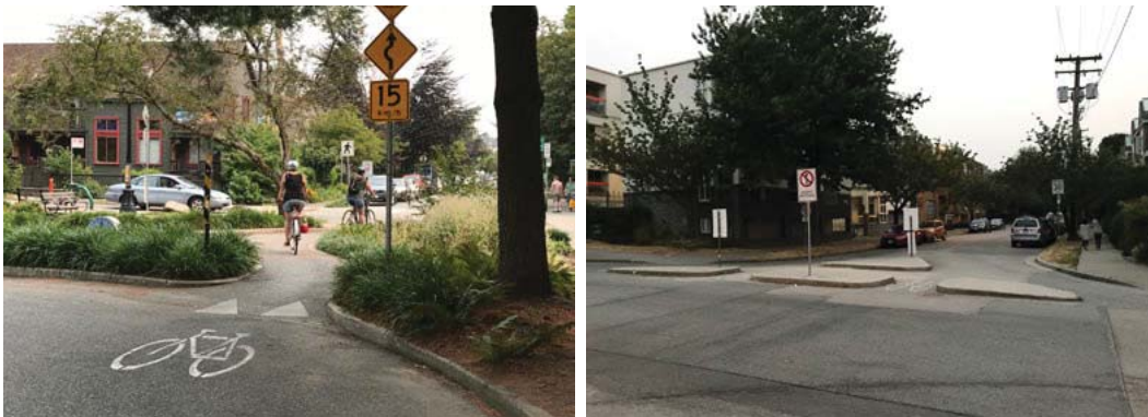
[Left] City of Vancouver – Neighbourhood Greenway with Road Closure for Motor Vehicles [Right] City of Vancouver – Neighbourhood Greenway with Right in/Right Out for Motor Vehicles
