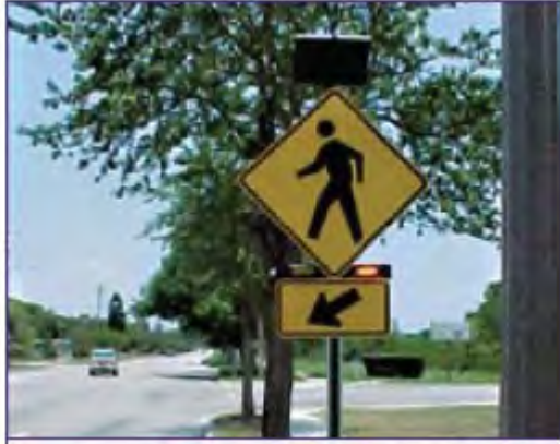
Figure 1 Roadside RRFB (FHWA)
