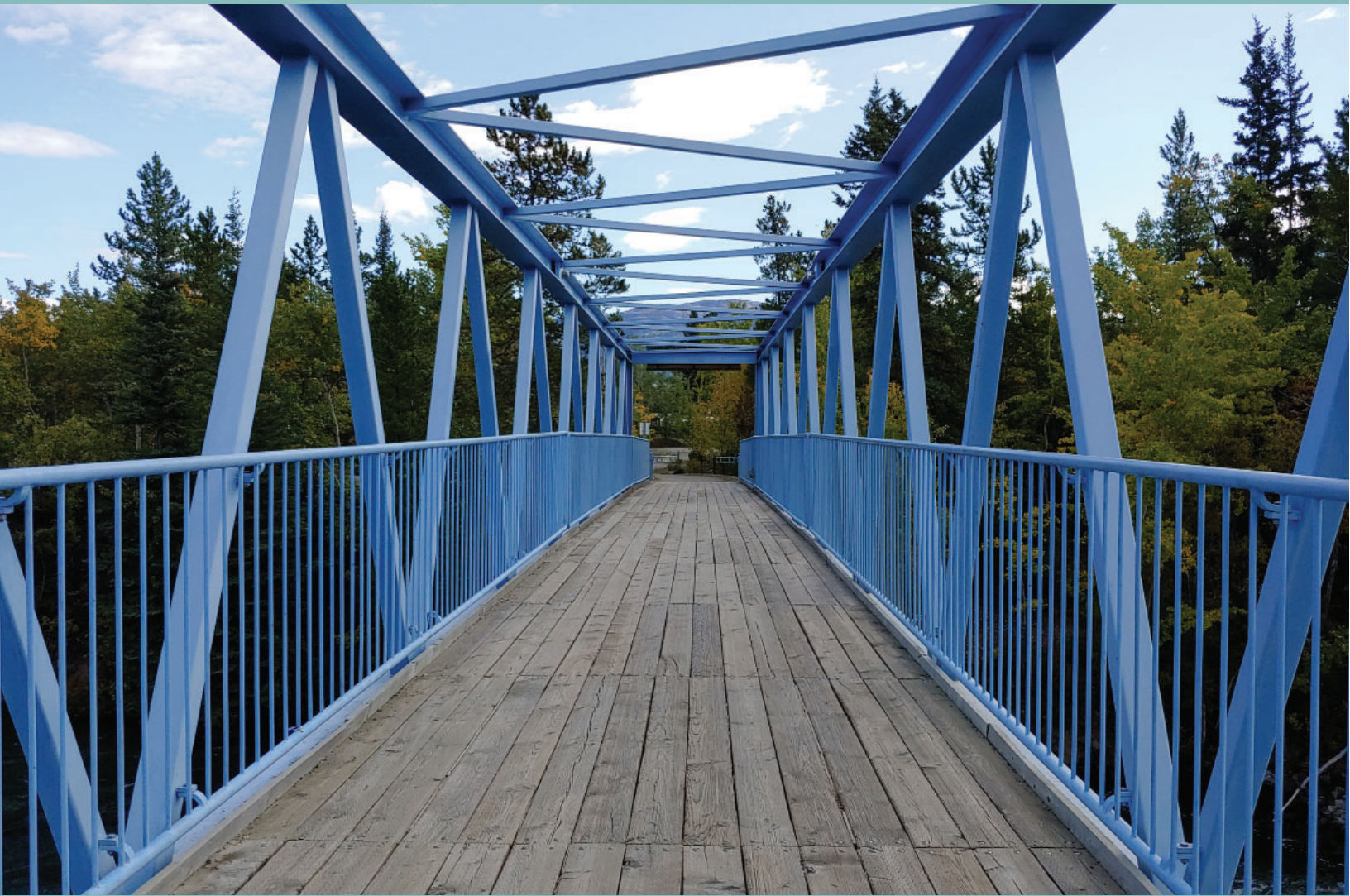
Figure 8 Rotary Centennial Bridge on the Millennium Trail
