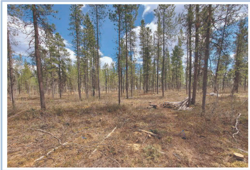
Photograph 10: areas have been cleared, with stacked log piles seen on the Subject Site (June 3, 2022)
