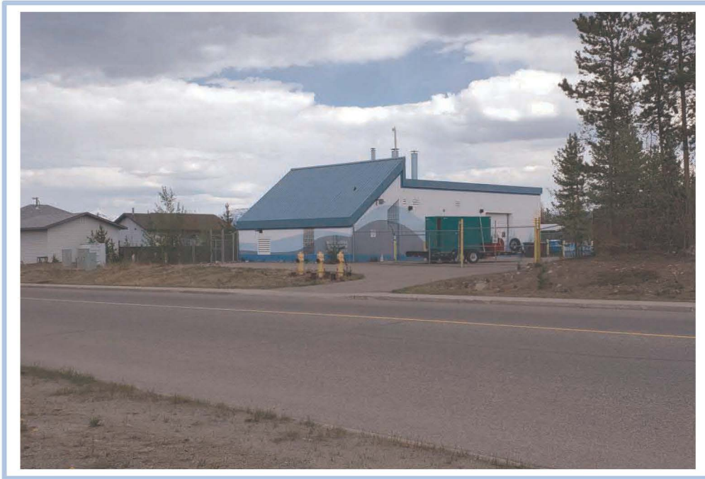
Photograph 1: Pump house located on Falcon Drive to the south of the Subject Site (looking southeast) (June 3, 2022).
