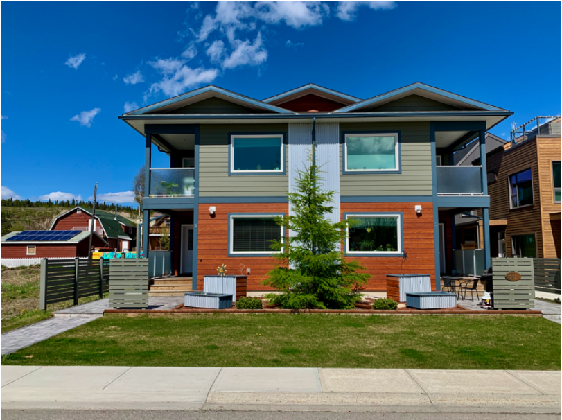
PHOTO 3: NEW MULTI-UNIT DEVELOPMENT DOWNTOWN BUILT ON PREVIOUSLY VACANT LOT (608 JARVIS STREET, RD)
