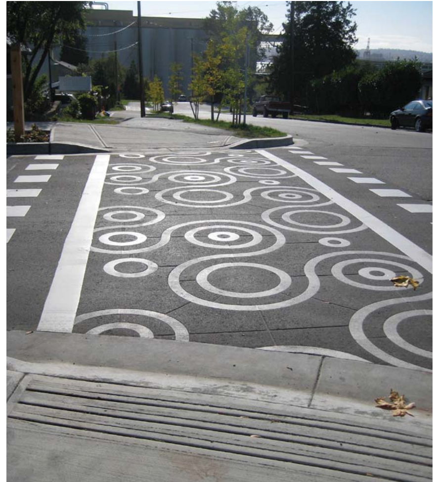
Spirit Trail crosswalk treatment (North Vancouver, BC)
