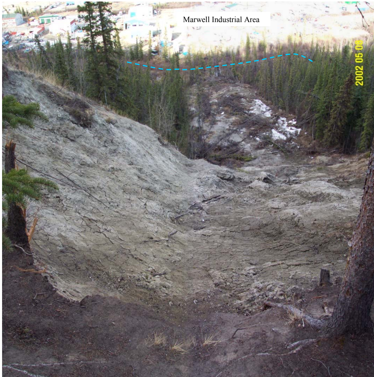
Photograph 10: May 2002. The Takhini debris slide, which occurred in July 2000, is located on the escarpment that separates the Takhini subdivision from the Marwell Industrial Area. It occurred behind the Northern Windows assembly plant on Copper Road. The toe of the deposition zone is close to a stream channel / drainage ditch (blue) and is within 50 m of private property.
