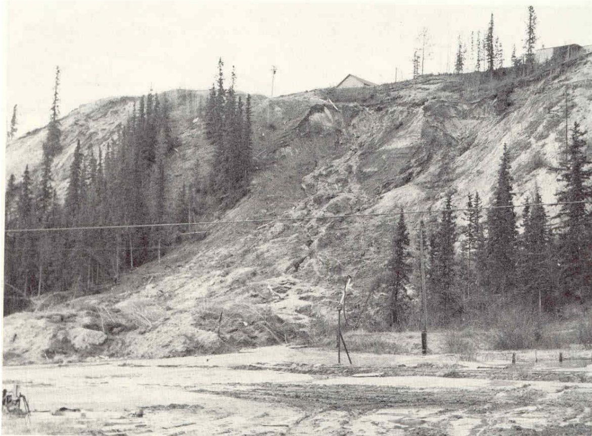
Photograph 2. [June] 1953. Landslide near Hoge Street (R.F. Legget).
