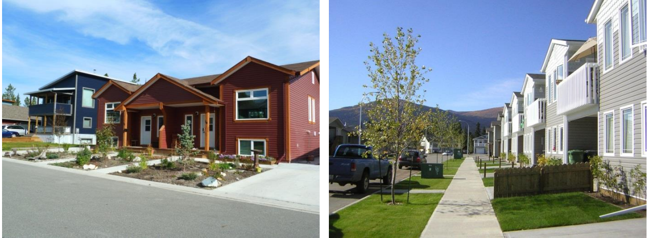
Figure 21: Landscape requirements and opportunities. Left: comprehensive landscaping in Takhini North. Right: boulevard planting in Porter Creek.
