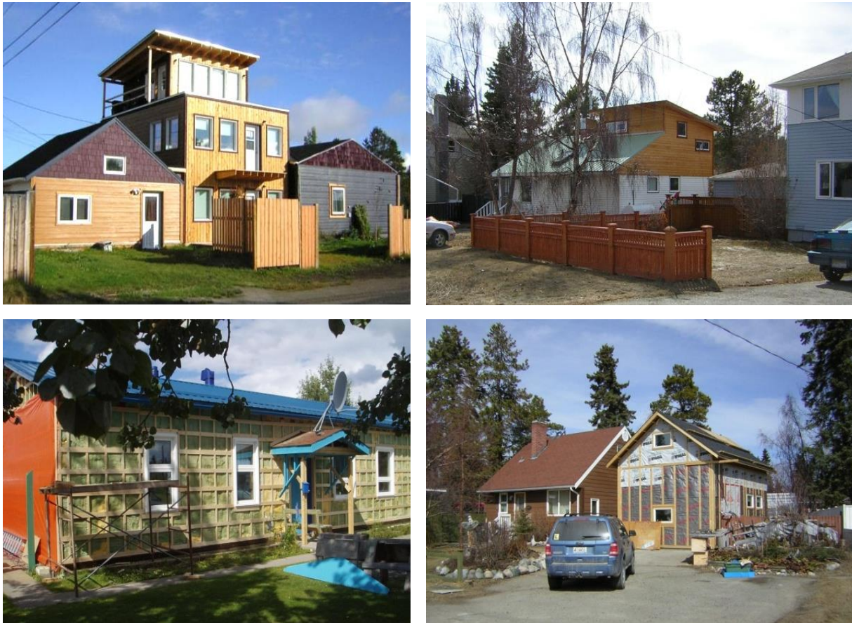
Figure 3: Renovations in Hillcrest. Clockwise from top left: SteeloX addition facing Hillcrest Drive; adaptive expansion on Klwane Crescent; garage addition on Klwane Crescent; energy-efficiency retrofit on Dalton Trail.
