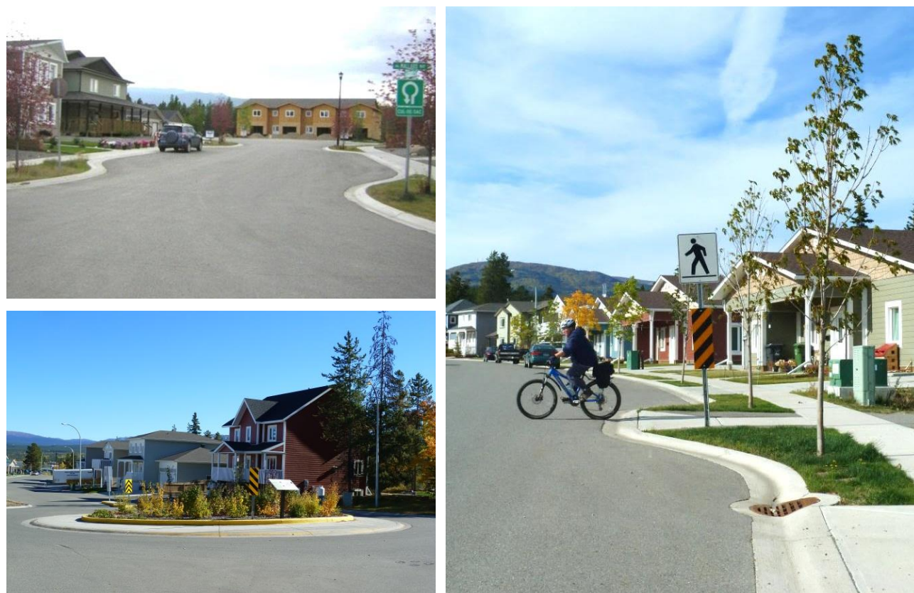
Figure 14: Potential traffic calming measures. Clockwise from top left: chicanes in Ingram; pinched crossing in Takhini North; roundabout in Takhini North.
