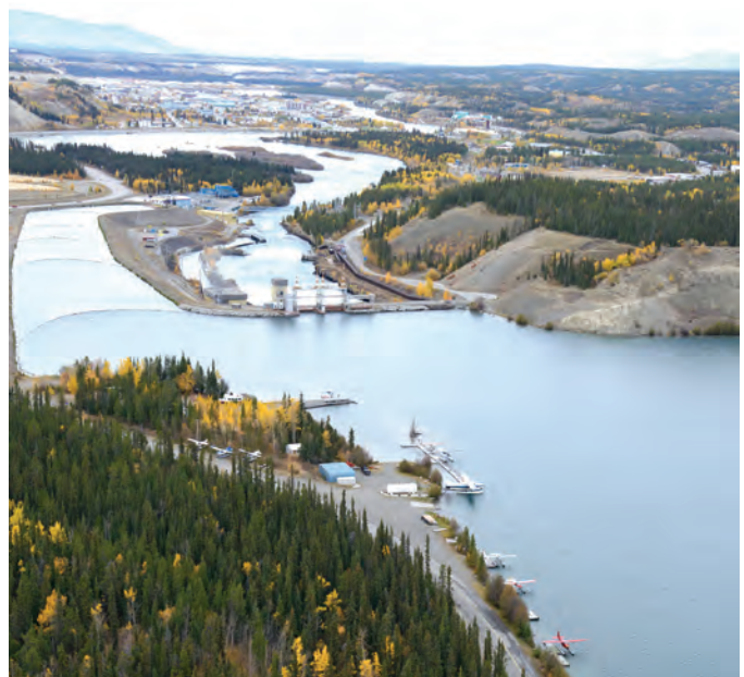
Aerial view of Lots 400, 401, and 402 near the hydro-electric dam
