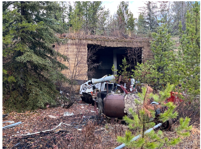
Concrete bunker on Lot 426
