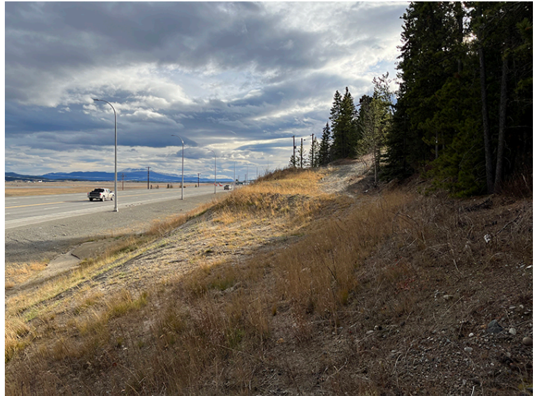
Looking south along the toe of TKC C-30B's steep slope
