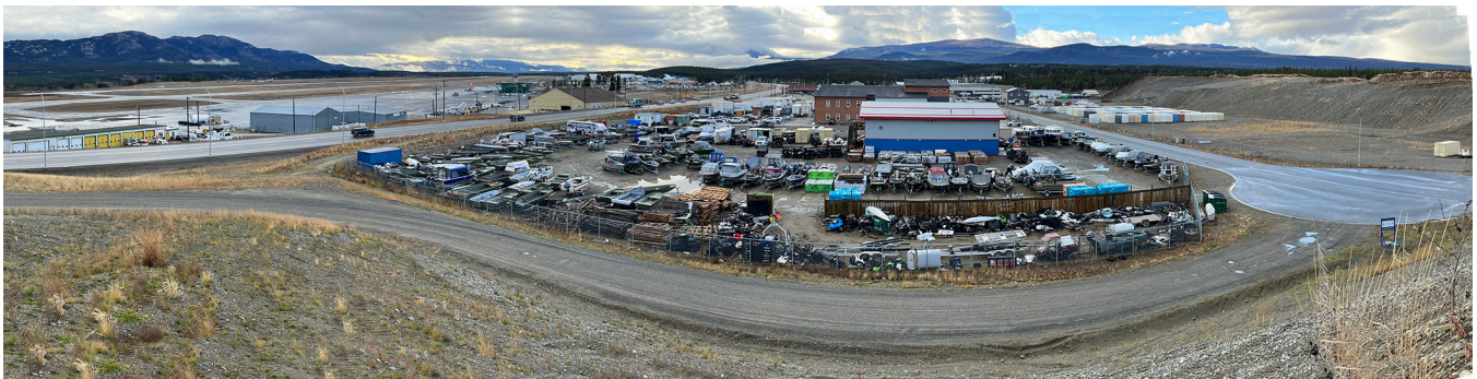
Panoramic view of Wasson Place from Lot 426
