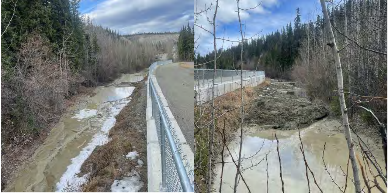
Photos 1 and 2: Existing Sediment Basin Looking North and South, Respectively
