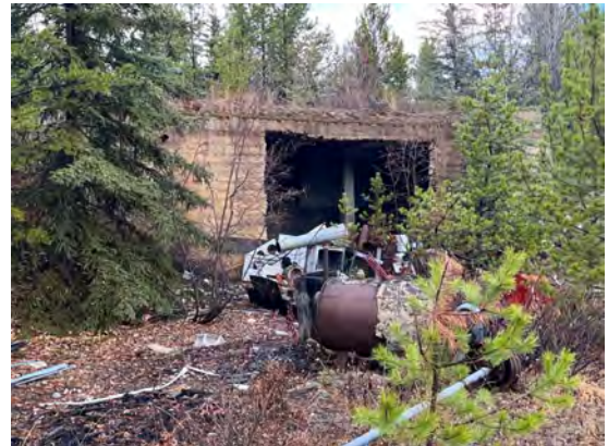
Concrete bunker on Lot 426
