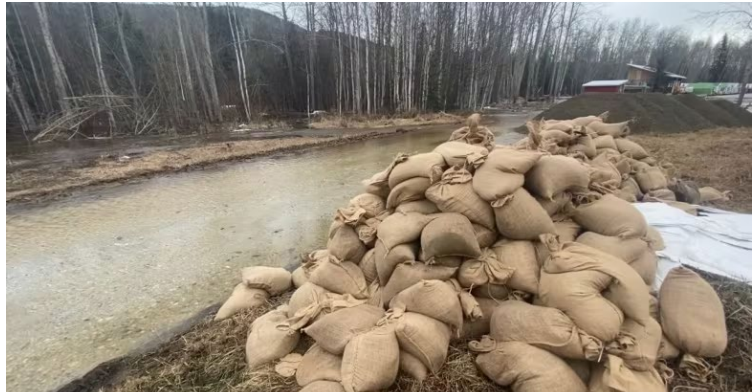
Figure 6 Sandbags to Mitigate Flood Waters
