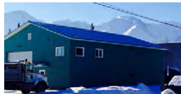
Water Truck Garage
