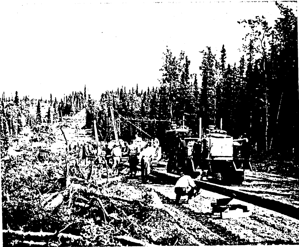
Construction of the Haines-Fairbanks military pipeline, 1954.
