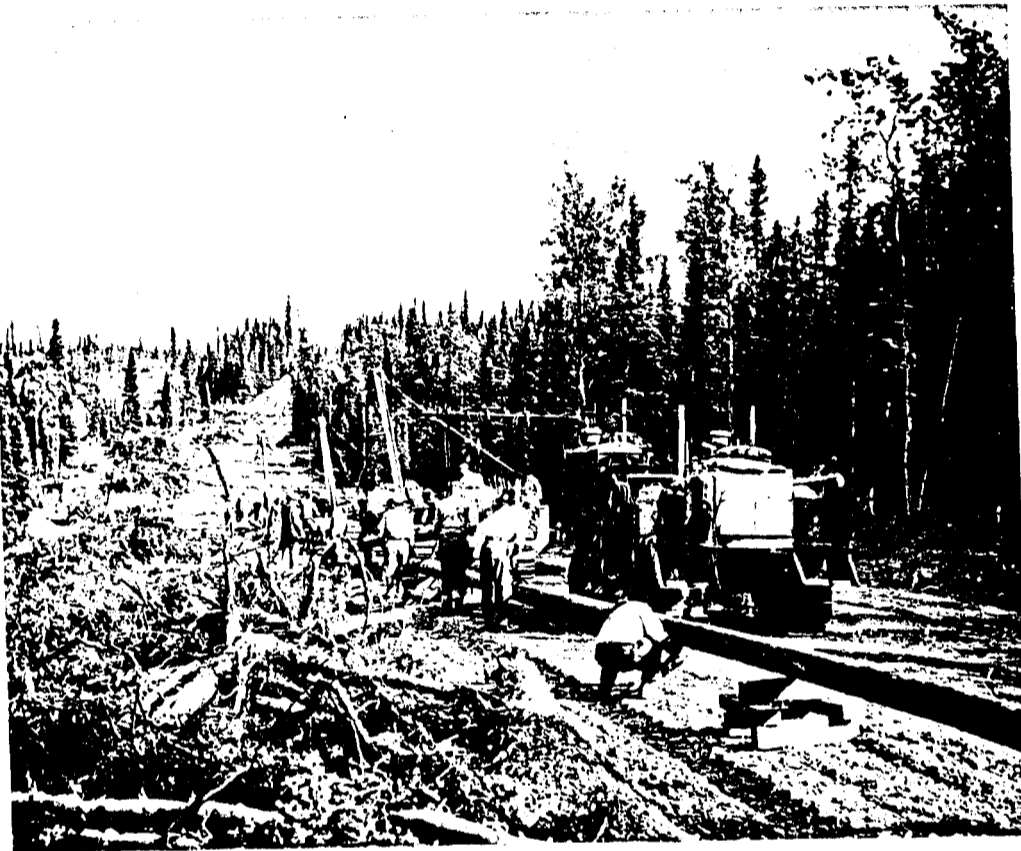
Construction of the Haines-Fairbanks military pipeline, 1954.
