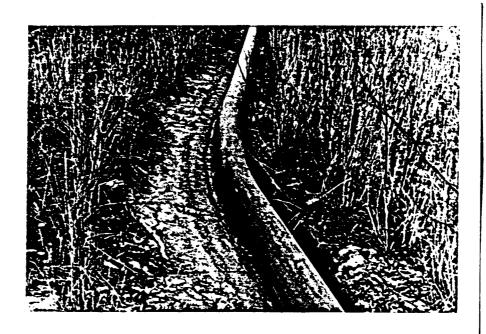
Line movement such as is shown in the above photo contributes to pitting if the soil conditions are favorable for corrosion. A slight film of rust removed from the pipe is shown below and adjacent to the left hand side of the pipe. No excessive corrosion was noted in this particular area.
