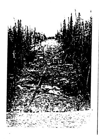
Soil conditions in this stream crossing at Mile Post 122.8 are generally gravelly in nature. It is doubtful that the waters of this particular stream are corrosive. A short section of line found imbedded in the gravels below the flowing water showed little or no deterioration.
