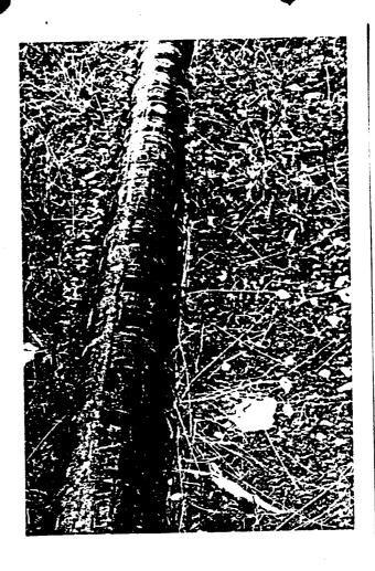
This picture taken at Pipe Line Mile Post 120.5 demonstrates areas that may corrode under favorable conditions. These are areas where the handling and/or manufacturing of the English steel shows removal of the original protective varnish. Areas similar to this are shown in Photos 1, 2 and 4 and under the environmental conditions are highly susceptible to concentrated corrosion.
