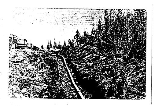
The above photo shows the uncovered petroleum line from approximate Mile Post 119.7 to Mile Post 119.11. This section of the line contains many localized areas of corrosion. The corroded areas were concentrated where varnish has been removed from the original pipe and where fine grain soils existed adjacent to the pipe.
