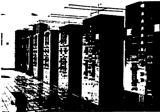
Bank of 7 RCA AT3 - 300 Watt Transmitters and one RCA 260B 2 Kilowatt Transmitter. Whitehorse communications building - 1942
