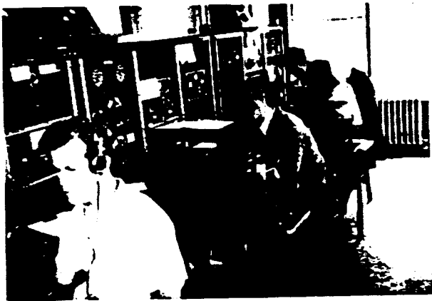
Whitehorse Radio Range Station - 1944 All three "positions" in operation. Operators: Bob Williamson, Russ Travers and two other operators busy at the Radio Range monitoring position
