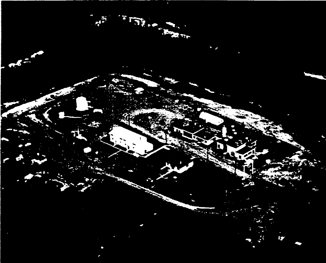
Donjek Pump Station, approximately 5 acres in area, is located 25 miles northwest of the trading post of Burwash Landing
