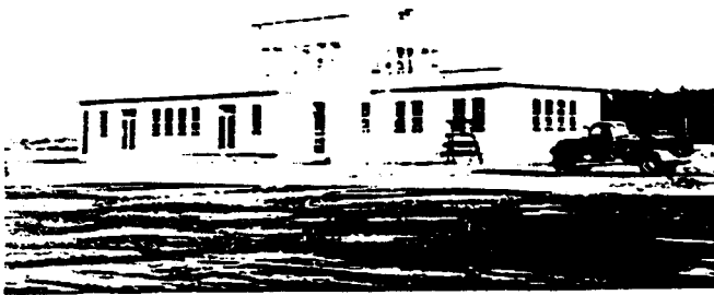
Whitehorse Airport Administration Building 1942 Where the Airport, Radio Range and Metrological offices were.
