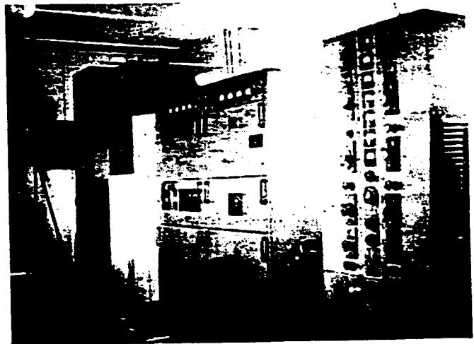
TYPICAL COMMUNICATION TRANSMITTERS AT AN INTERMEDIATE STATION Centre - AG500 4-channel 500 Watt Transmitter and a 2-channel AT3 300 Watt Transmitter
