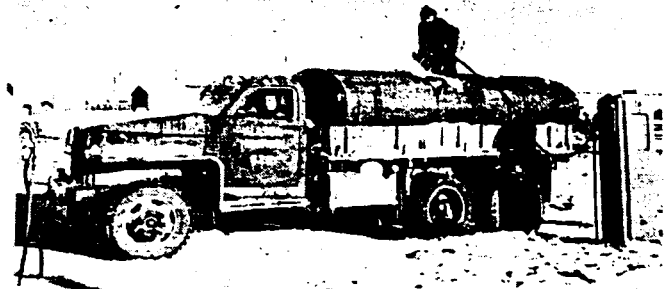
MANY THOUSANDS of gallons of petroleum products were hauled by the Studebaker 6x6 1500-gallon tankers, to supplement the pipeline deliveries.
