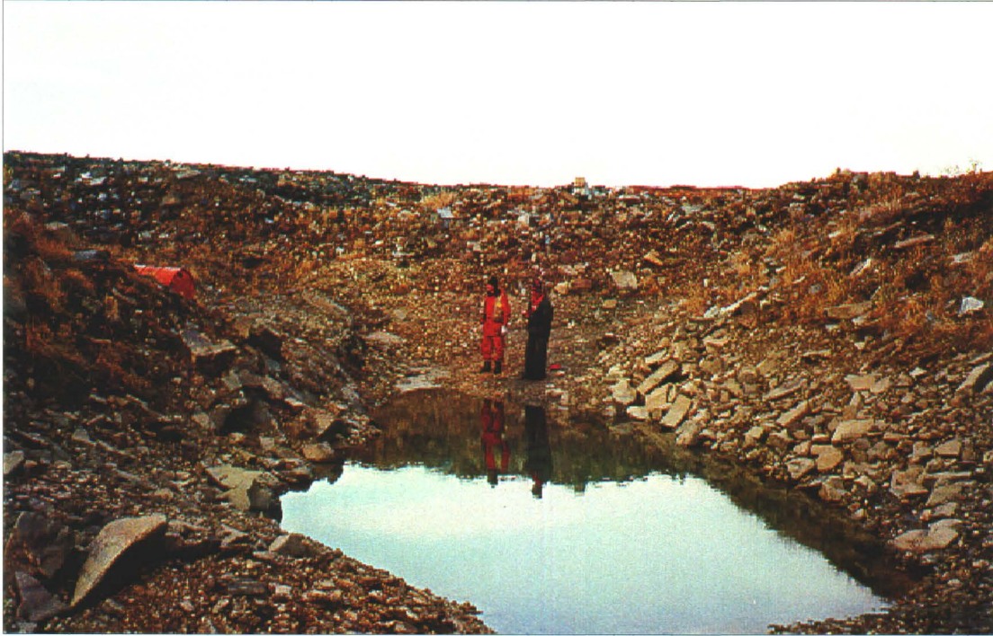
Photo 38-1 : Fox. Water ponded at the base of Trench #1. (Azimuth 020 o )
