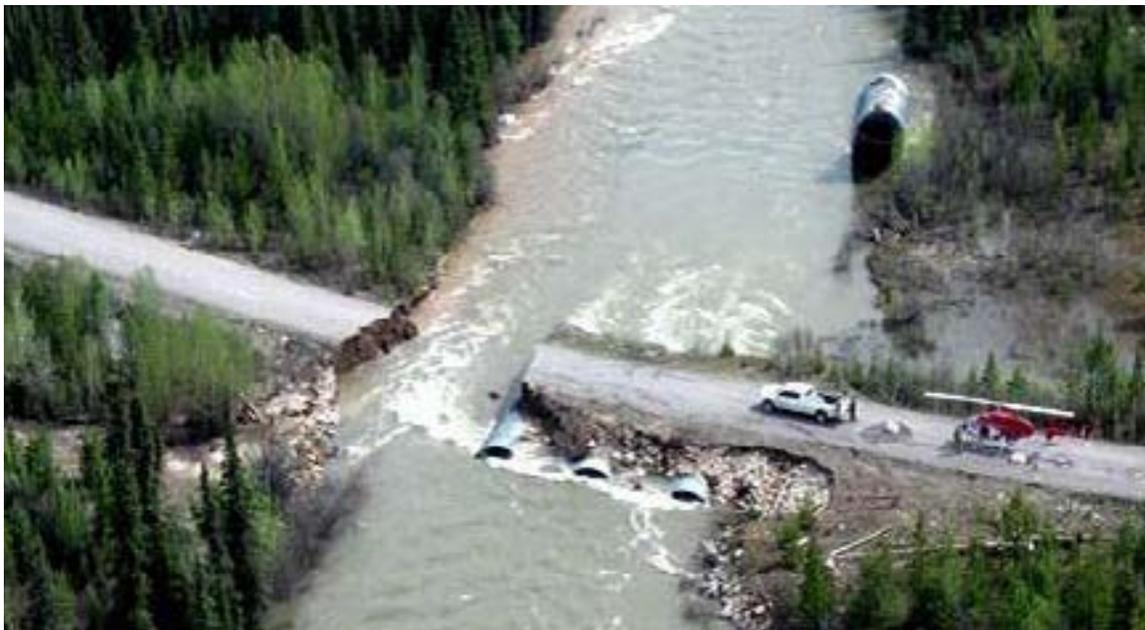
**Figure 6.** The Nahanni Range Road, which leads to the mine, was washed out in three locations; however, the culverts displayed no obvious corrosion or deformation (Yukon Department of Highways and Public Works).
