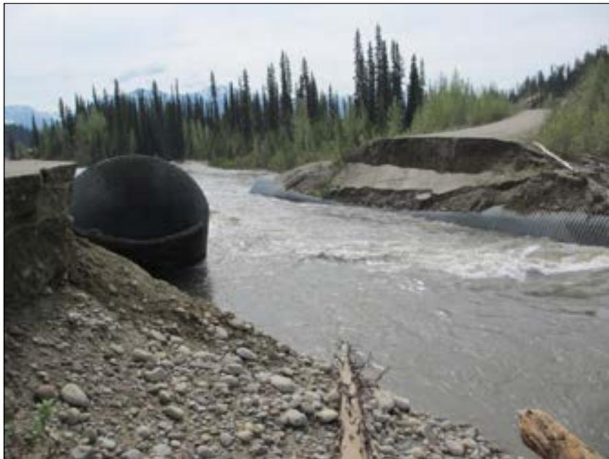
**Figure 1.** Washed out culvert on the Nahanni Range Road #1 (June 2012).
