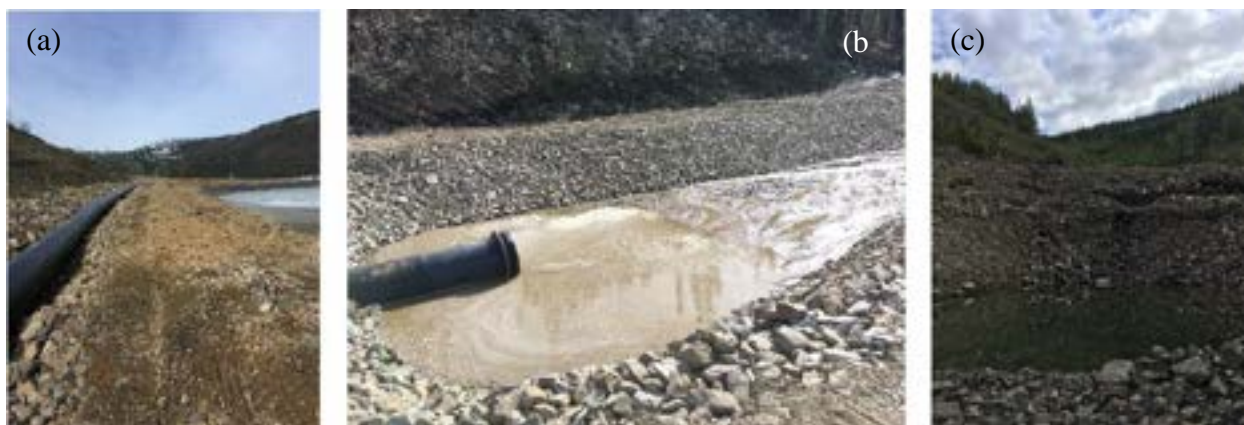
Figure 3: MCW sampling locations: (a) pipe exit near the treatment pond; (b) the pipe entrance at the Platinum Gulch Waste Rock pile, and (c) the pond above ditch A.
