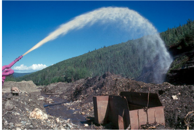
Figure 9: Monitoring of ice-rich ground, Klondike area. There is no containment method being used, allowing sediment and organic material to enter the creek directly.
