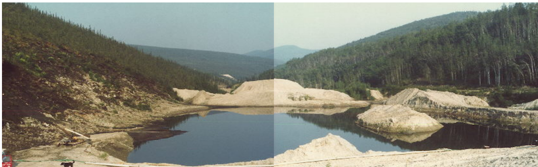
Figure 10: View down Upper Bonanza Creek, showing a well-constructed, large volume settling pond. Sediment input is from the left, as indicated by the well-developed fan. Permafrost is present on the north-facing slope (left), and absent on the south-facing slope (right).
