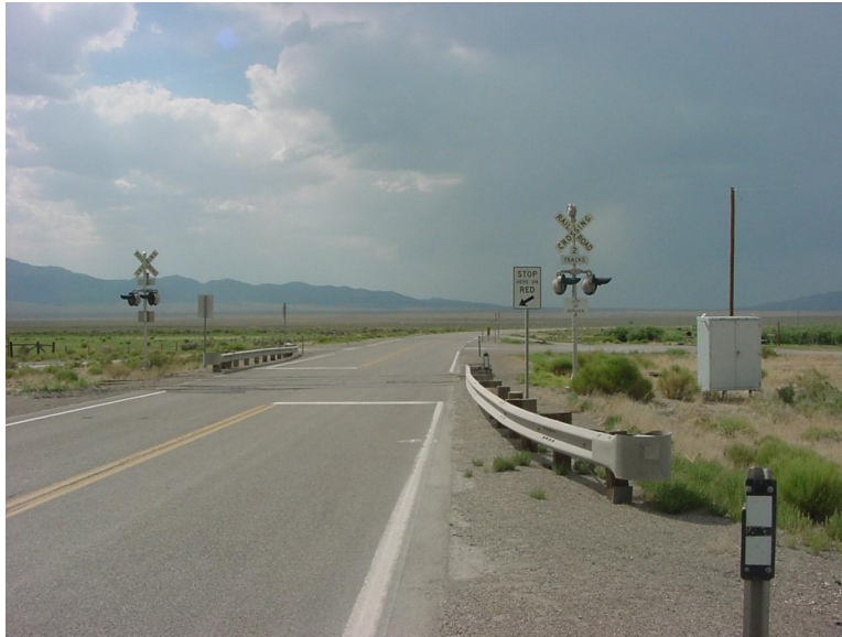
Picture 20: Level Road Crossing
