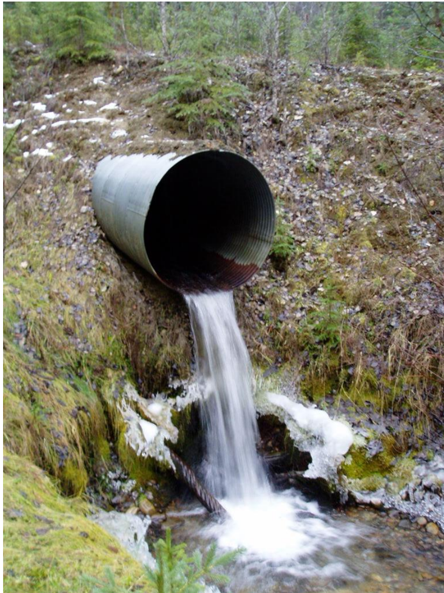
Picture 19: Bridge Pipe
