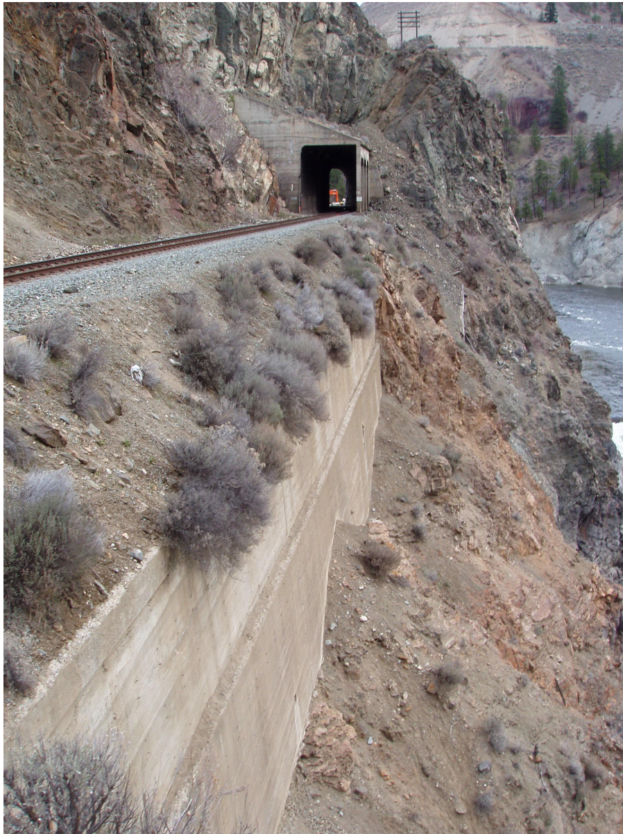
Picture 28: Concrete Retaining Wall
