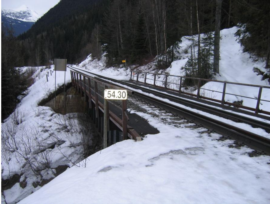
Picture 17: Small Bridge over Tributary
