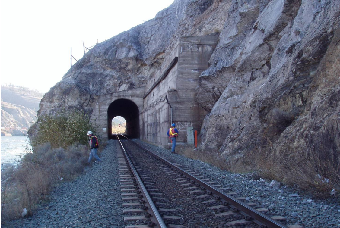
Picture 16: Short Tunnel and Buttress at Portal
