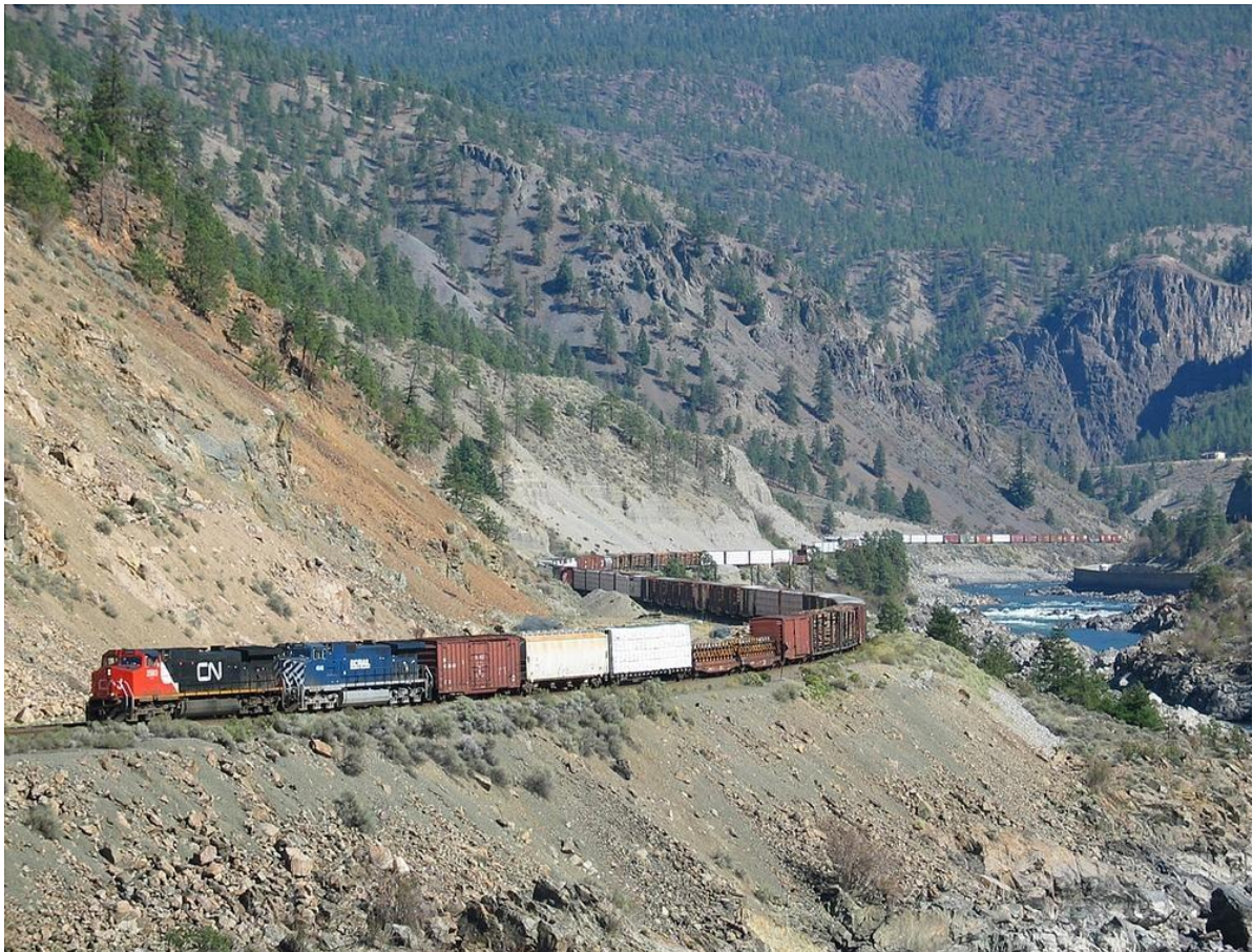
Picture 14: Very Heavy Grade Construction
