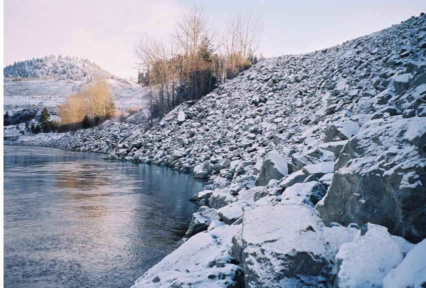
Picture 22: Riprap Erosion Protection
