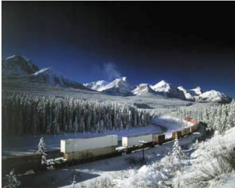
Picture 13: Heavy Grade Construction
