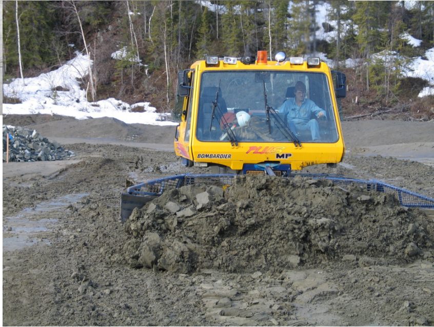
Surface re-grading was performed using a snow cat
