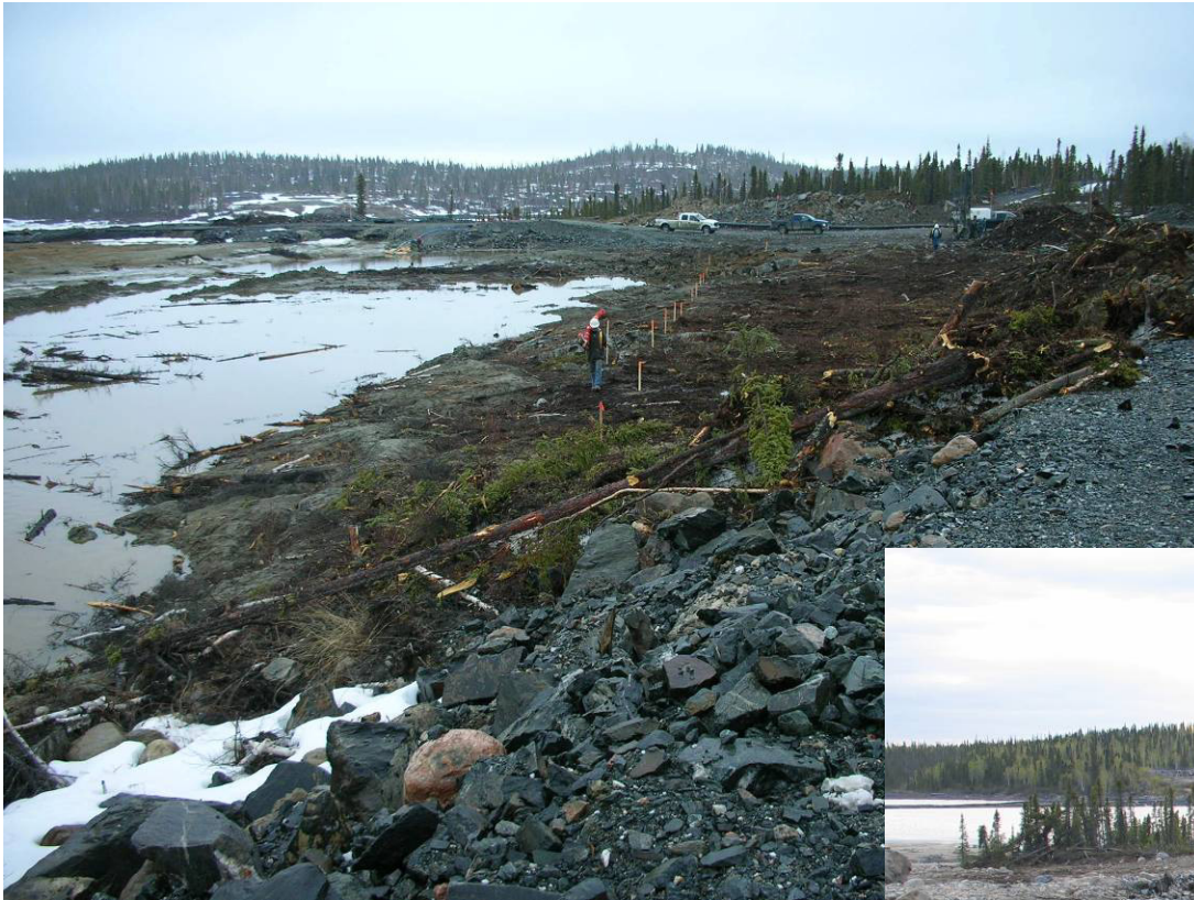
Start of Dyke 7 Spillway excavation with excavation and blasting of bedrock
