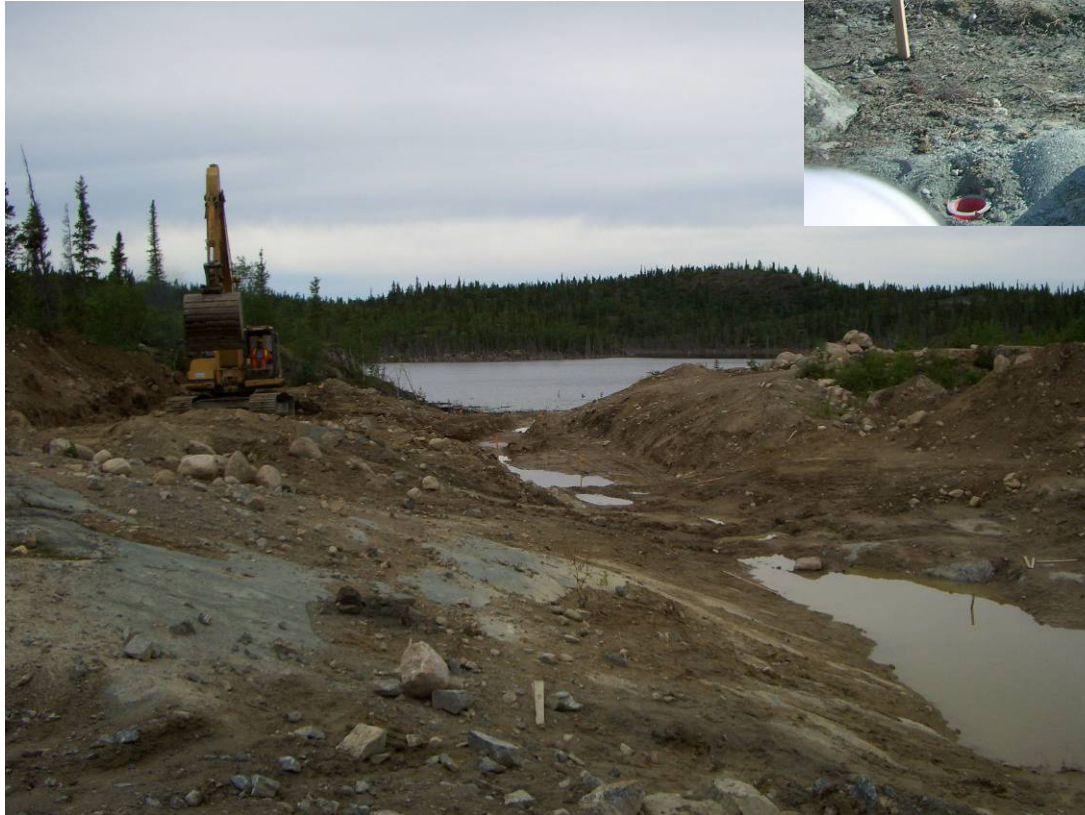
Excavation of till along the upstream reach of the Discharge Channel
