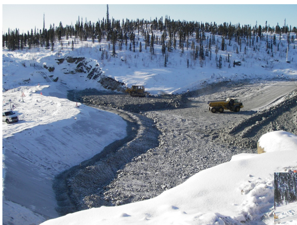
Completion of the infill between Dam 1 and Dam 1B
