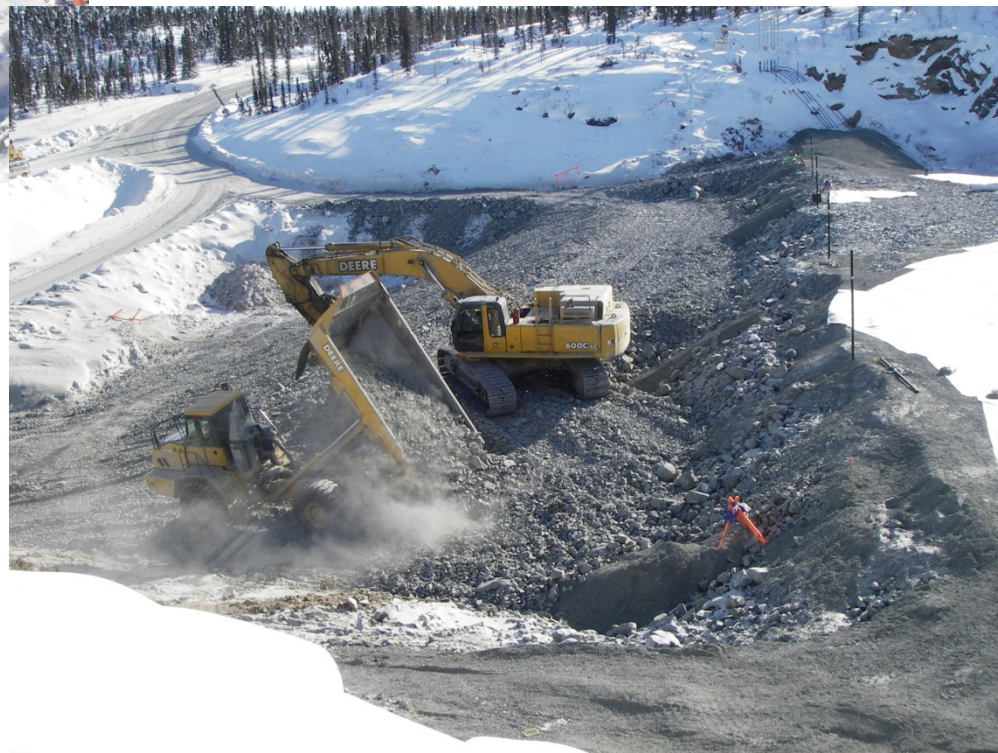
Completion of the downstream face of Dam 1B
