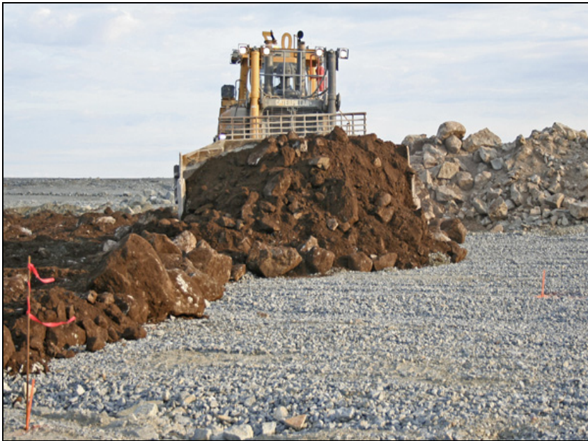
Spreading topsoil topdressing
