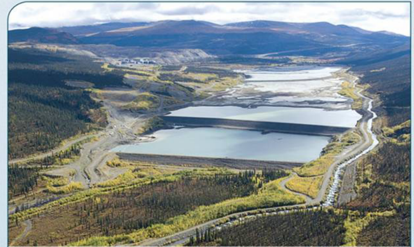
Before remediation (Now)
