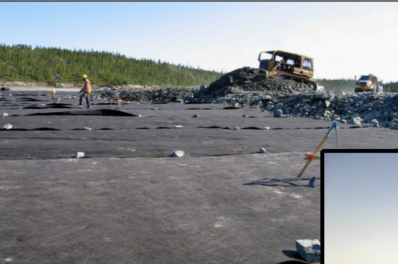
Placing cover on geotextile.
