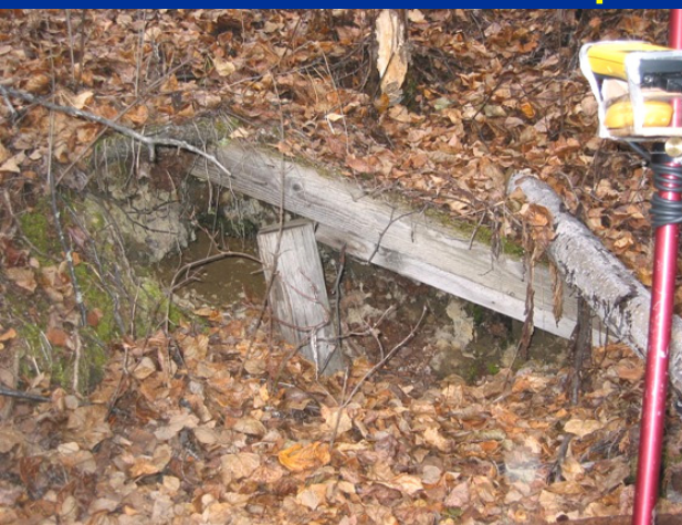
Collapsed Portals along RR grade
