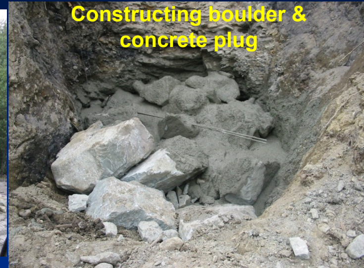
Large-dimension fill atop concrete plug
