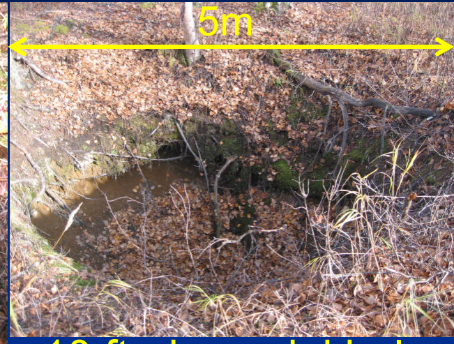
10 ft. deep sinkhole above Eska adits
