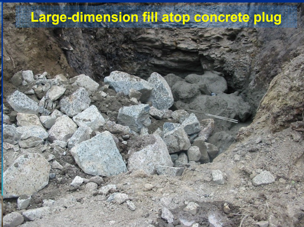
2 nd course of boulders, concrete, & rebar
