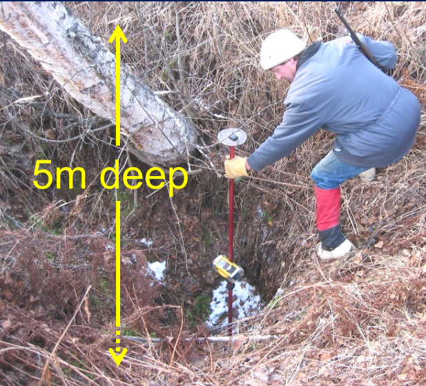
Conic subsidence pit
