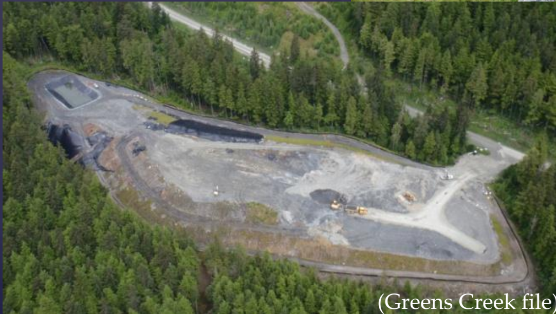
View of Greens Creek waste rock pile removal (left) and replacement of pyritic rock with non-pyritic fill (upper right)
