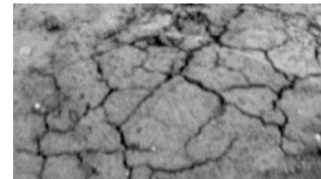
Surface cracks in tailings cover
