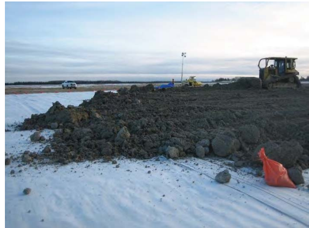
Figure 5. Clay being applied over the GCL.
