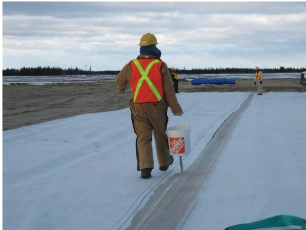
Figure 4. Spreading of loose bentonite between GCL sheets to provide a continuous hydraulic seal.
