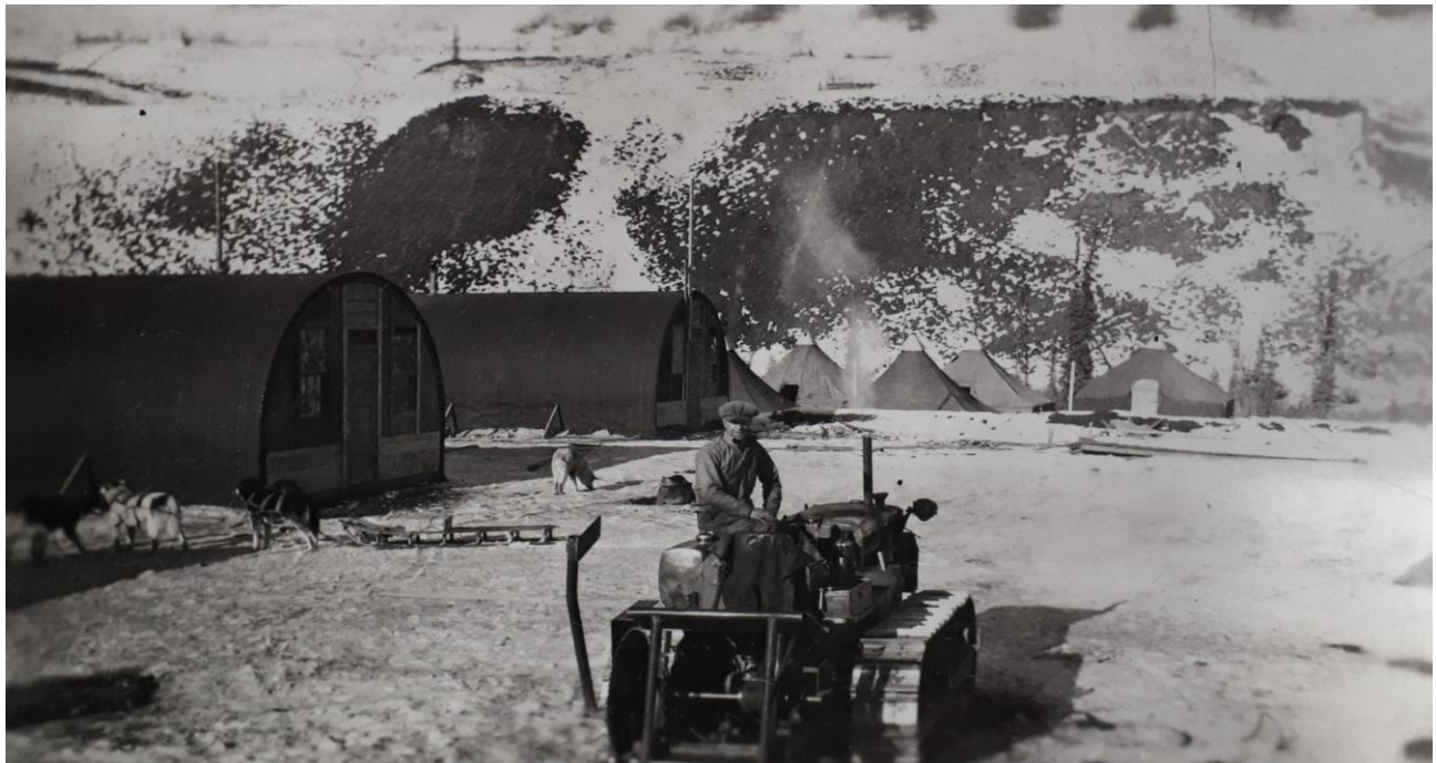
Canol construction camp at Ross River in 1942. Dorothy John fonds 92/17 #9 PHO 433
