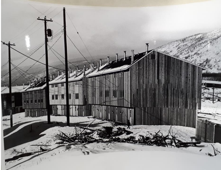
A typical maisonette, Faro 1970. The maisonettes received much criticism the first year. They had inadequate insulation and furnaces, the overhang was uninsulated, and the houses had only one exit. Yukon Archives, Richard Harrington fonds 79/27 #146 PHO 103.
