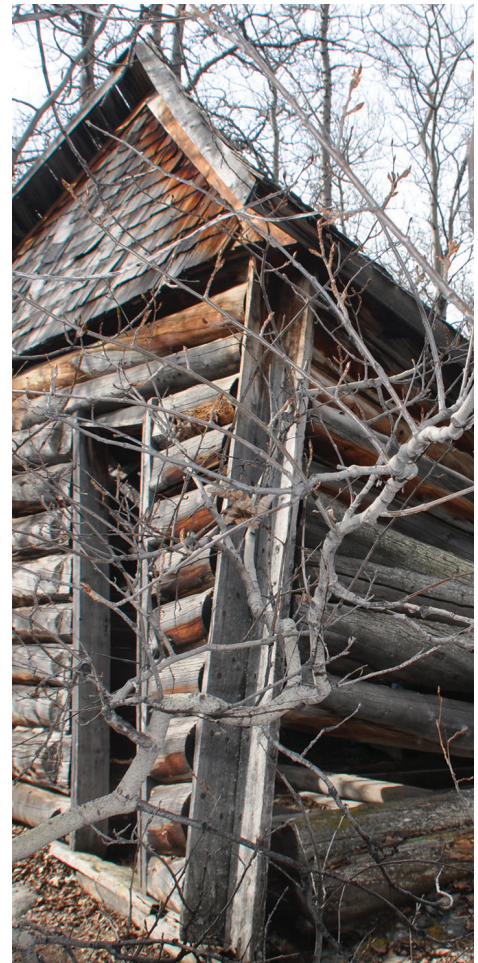
Example of a Yukon corner, Cabin 2.
