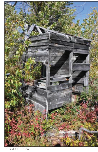
2017\DSC_0024 VIEW FROM THE SOUTHEAST NTS
