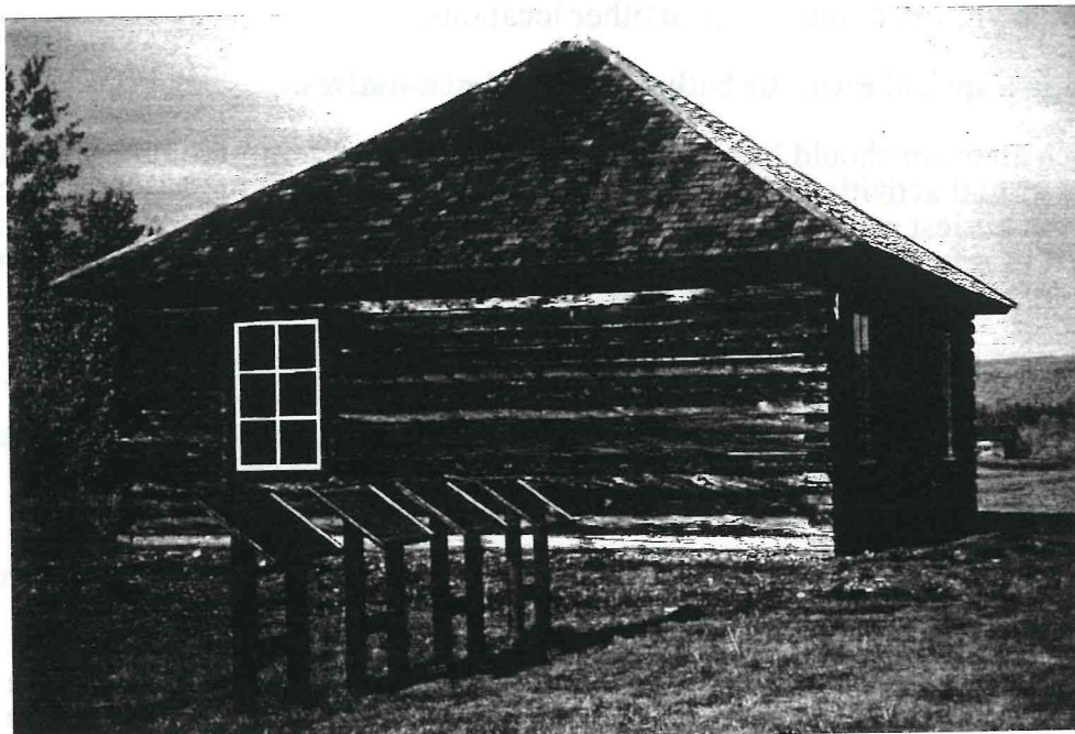
The restored Yukon Field Force orderlie's quarters with interpretive signs. Refer to interpretive framework for details on proposed sign plan.
