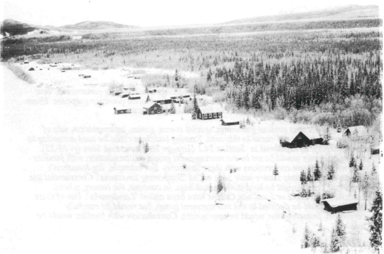
Fort Selkirk, looking south along the banks of the Yukon River. The campground and Drying Cabin is visible in the foreground, with the Stone House just to the right. This part of the site will be used mainly for visitor services and facilities. (J. Peepre, Dec. 1989)
