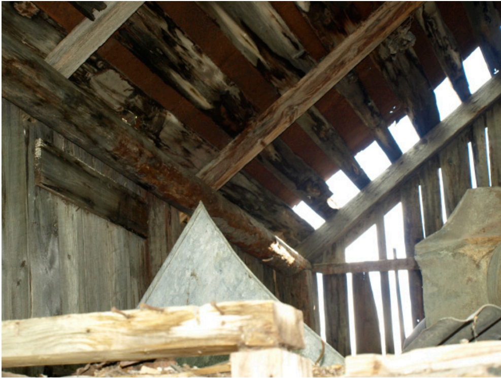
9. Interior Photo: Upper Floor
