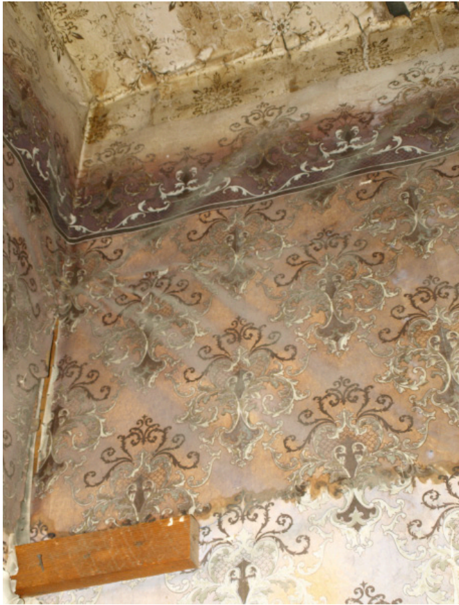
19. Interior Photo: Remaining Wallpaper
