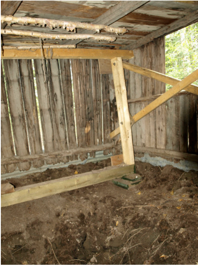
7. Interior Photo: Temporary foundation
