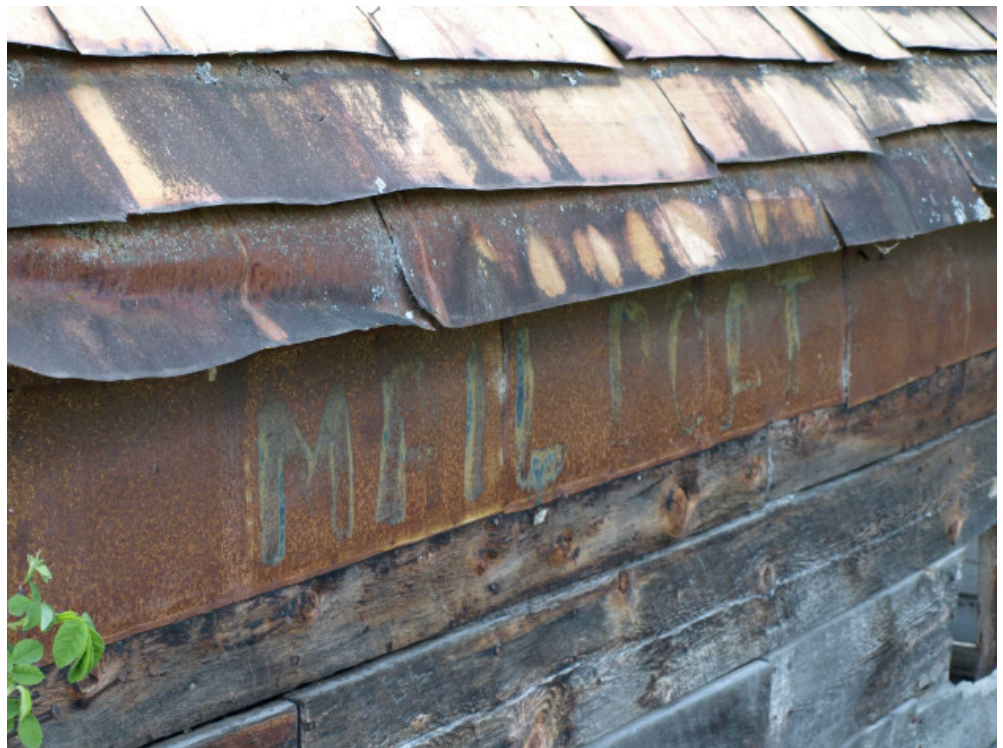
21. Exterior Photo: Roof Detail
