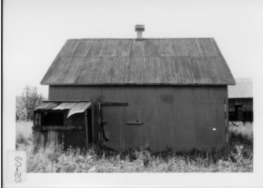
Photo: Waterway Survey Photo, 60-20
