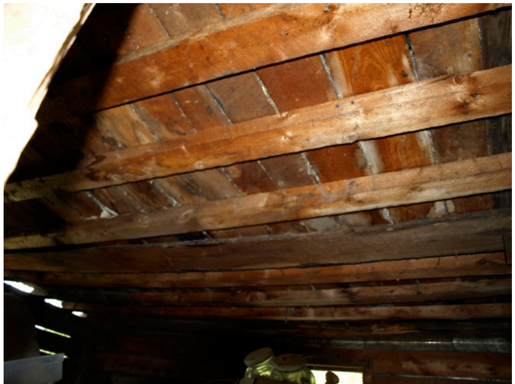
25. Interior Photo: Lower Floor Ceiling
