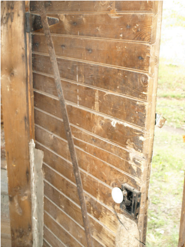
19. Interior Photo: Front Door
