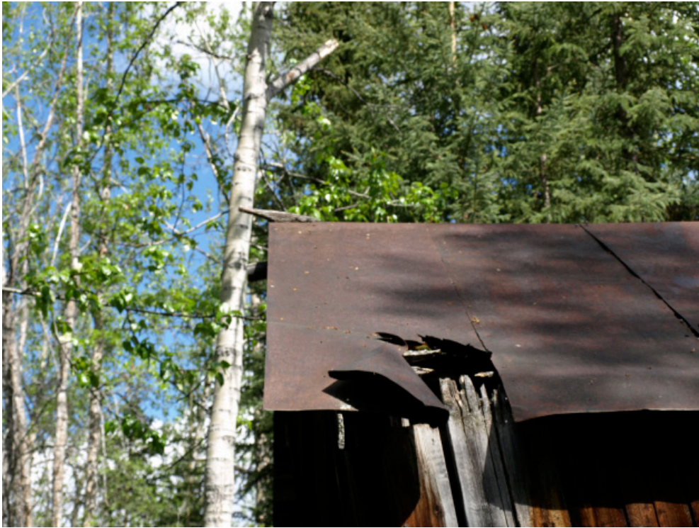
13. Exterior Photo: Detail photo of roof
