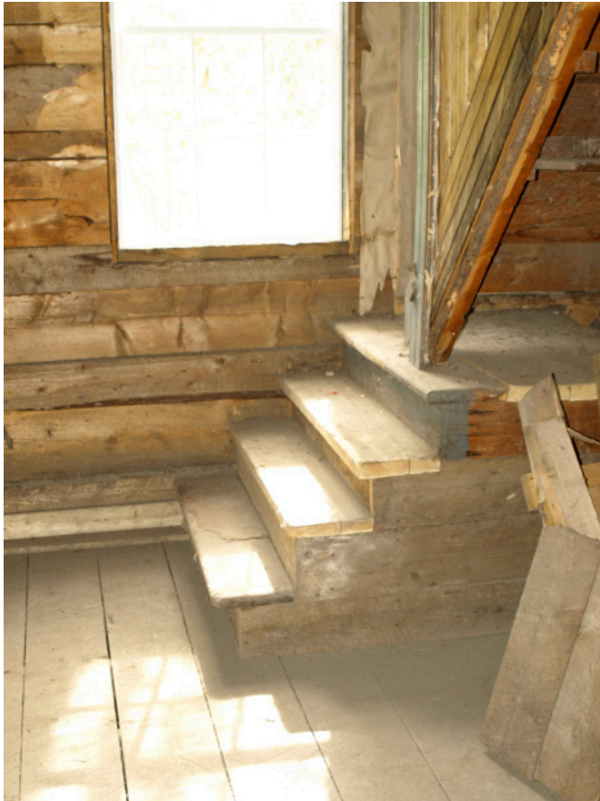
46. Interior Photo: Stair
