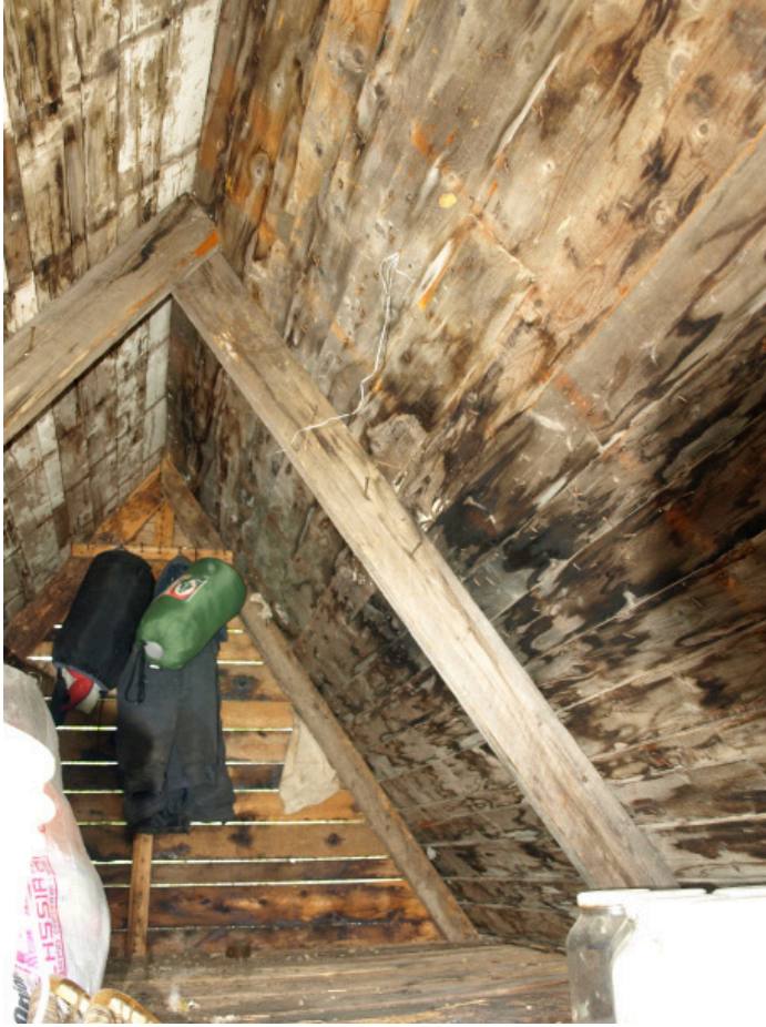
28. Interior Photo: Upper Floor
