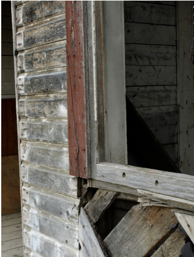
15. Exterior Window: Double pane window with venting holes.
