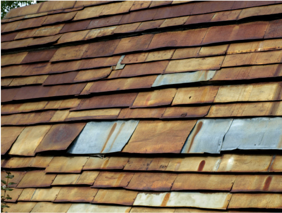
20. Exterior Photo: Roof Detail
