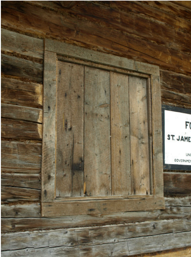
15. Exterior Photo: Window
