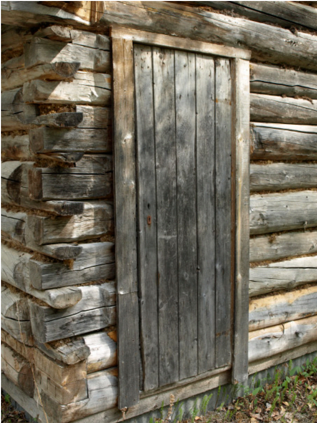
17. Exterior Photo: Rear Door
