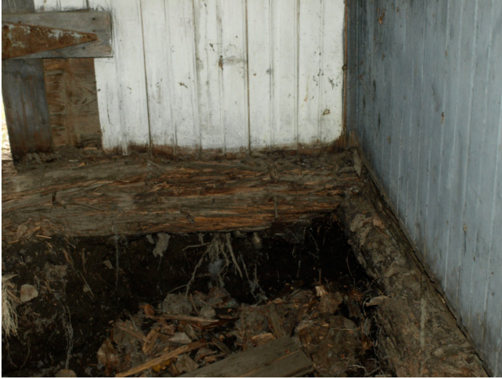
35. Interior Photo: rear shed
