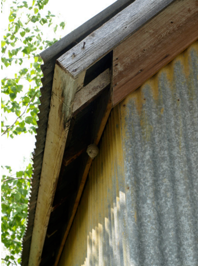
10. Eave Detail Photo
