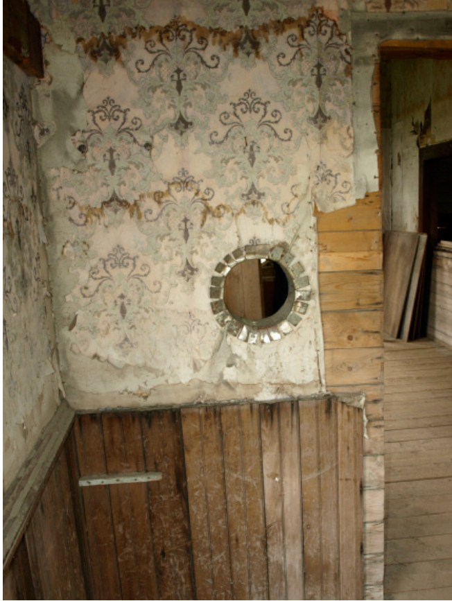
21. Interior Photo: Existing wood burning fire vent hole
