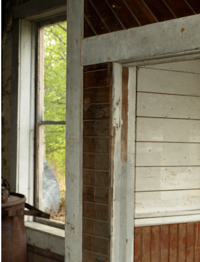
35. Interior Photo: Exterior Door/ Vestibule
