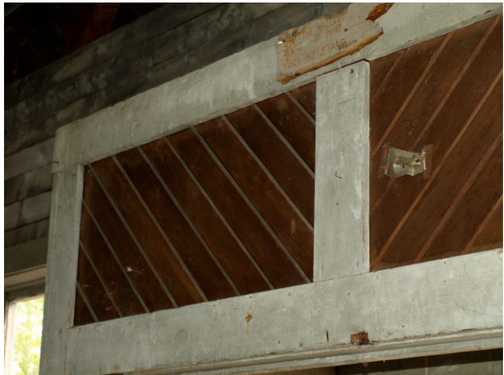
34. Interior Photo: Existing Transom Windows
