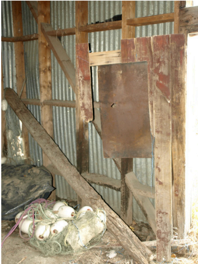
16. Interior Photo: Front Door remnants
