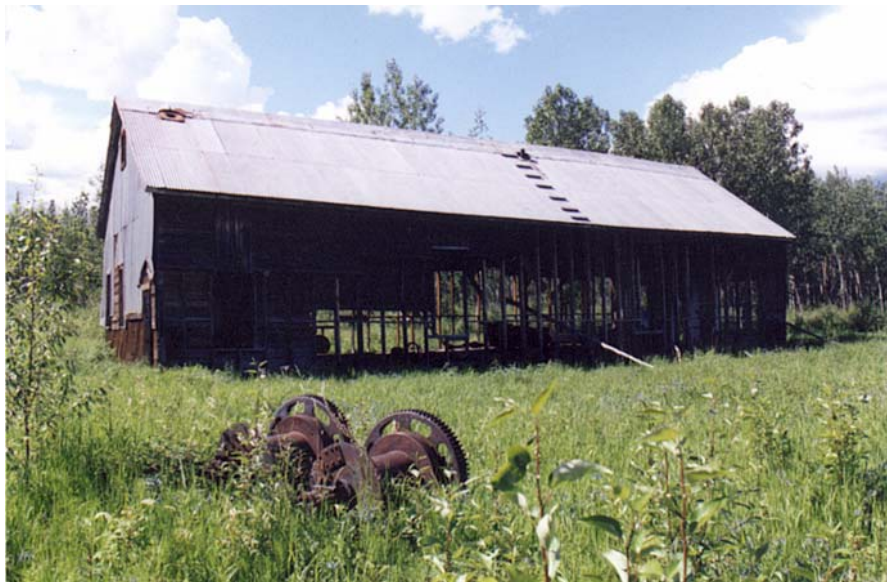
Appearance from North Side of Building, As Found Condition, June, 2002
