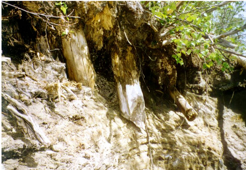
Fort Constantine: Remains of Palisade exposed due to erosion of the river bank, June 2002
