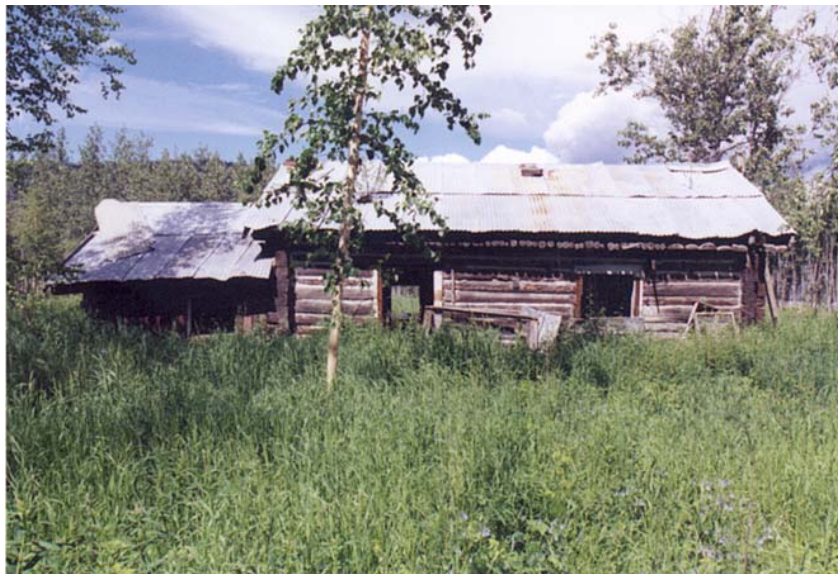
South Elevation, June 2002
