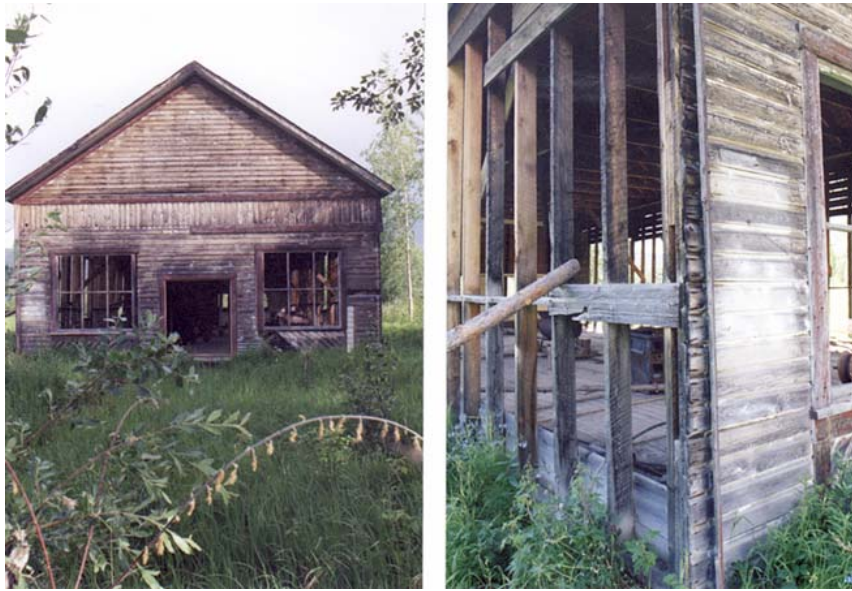
Northwest Elevation and North Corner, As Found Condition, June, 2002
