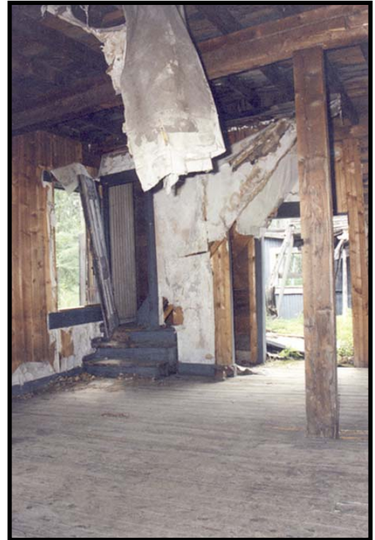
Figure 2.5: Building 12, North-West Mounted Police Building, Structural Collapse
