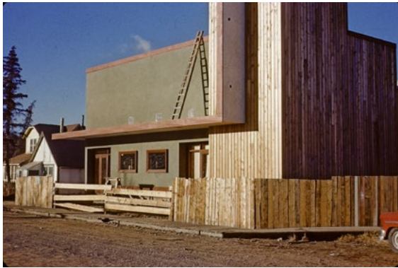
The Yukon Theatre under construction in 1954.
