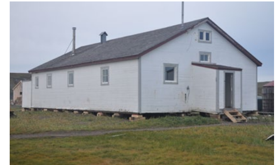
The Pacific Steam Whaling Co’s Community House before the lift in 2019 (top), and after the lift in 2023 (bottom).
