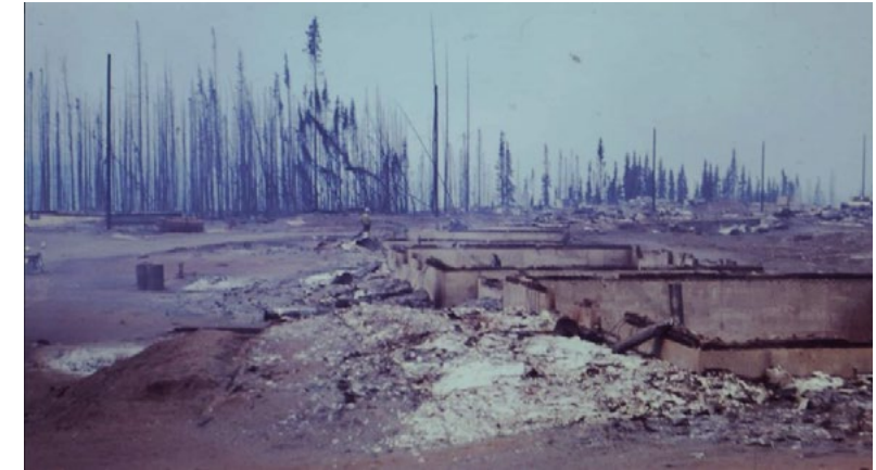
Following the lightning-caused fire in 1969, the town had to be rebuilt.
