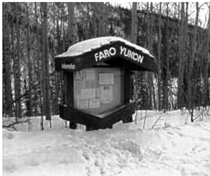
Protective roof effectively sheds snow from signage but parking area ploughing leaves berm, making it difficult to get close enough to read
