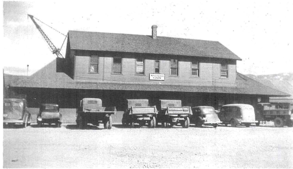
Figure 13. West elevation of depot before alterations, ca. 1942. YA, Preston coll., PHO 312, 78.
