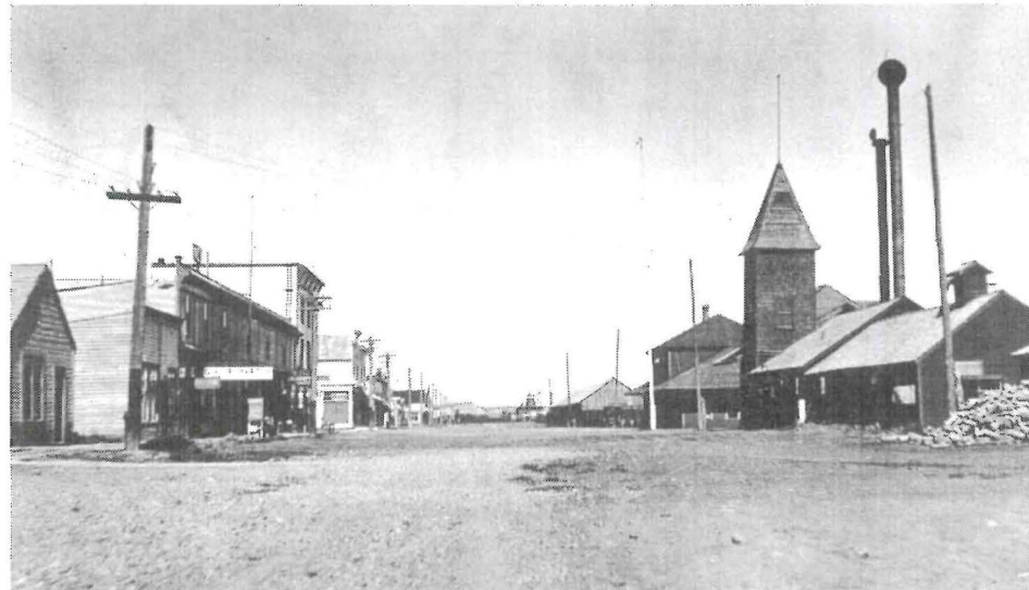
Figure 26. Looking north on Front St. YEC plant and firehall at right, n.d. YA, Hamacher coll., PHO 289, 50a.
