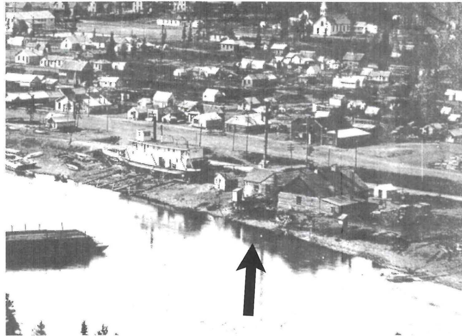
Figure 23. "Whitehorse after the fire, 23 May 1905." Taken looking southwest from across Yukon River. Note the boiler stack of the YEC building in its original location just south (right) of the Whitehorse Steam Laundry. Cropped from: YA/Old Log Church Museum coll., 79/107, PHO 117.
