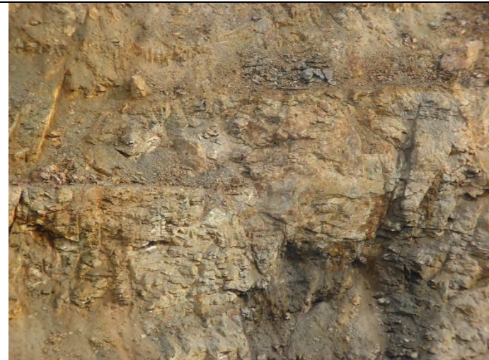
Photograph 36: Looking at Vangorda Pit side walls, showing rock raveling and slumping failures (2) – 09-10-2013
