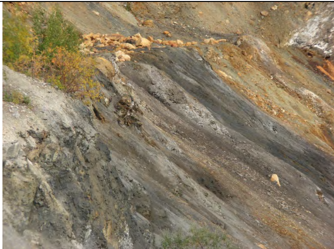
Photograph 39: Looking at Vangorda Pit side walls, showing rock raveling and slumping failures (5) – 09-10-2013
