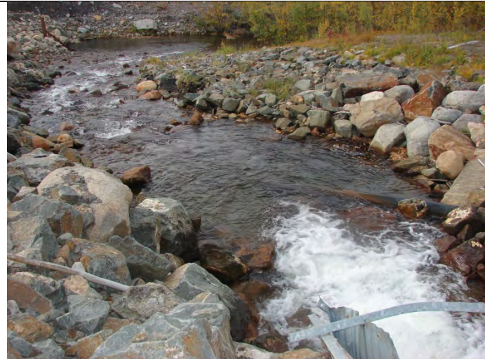
Photograph 2: Looking at the Plunge Pool from half-round 2,400 diameter CSP Culvert – 09-10-2013
