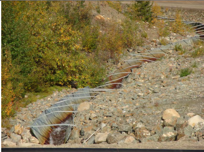
Photograph 9: Looking at the half-round 2,400 diameter CSP Culvert – 09-10-2013
