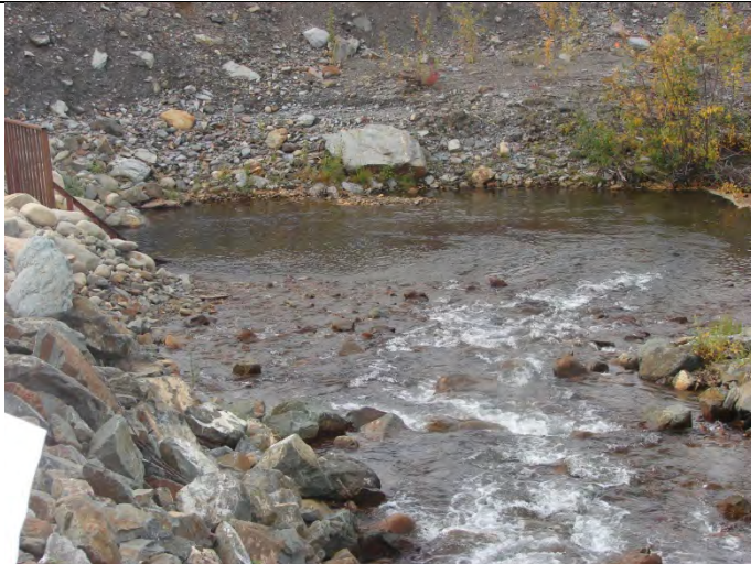
Photograph 1: Looking at VCD Plunge Pool – 09-10-2013
