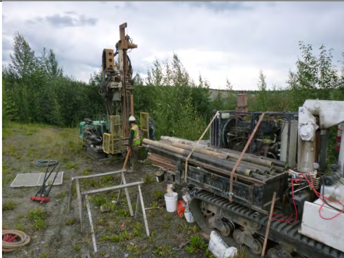
Photograph 41: Showing the set up for borehole CH13-303-BH001
