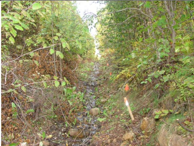
Photograph 21: Looking at the existing channel south of SRK proposed alignment, between station 0+900 and 1+000 – 09-10-2013
