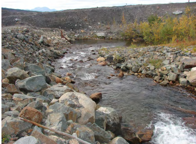
Photograph 3: Looking at the Plunge Pool from half-round 2,400 diameter CSP Culvert – 09-10-2013
