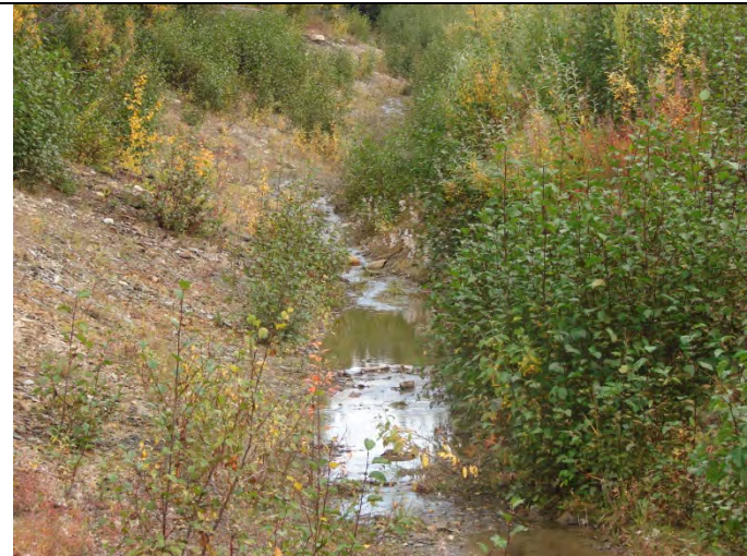
Photograph 24: Looking at the existing channel south of SRK proposed alignment, between station 0+600 and 0+800 (1) – 09-10-2013
