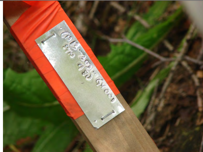
Photograph 22: Looking at the existing channel south of SRK proposed alignment, close to Geophysical Survey station marker CH13-303-GX001 – 09-10-2013
