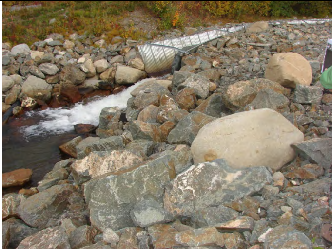
Photograph 5: Looking at the downstream of half-round 2,400 diameter CSP Culvert – 09-10-2013
