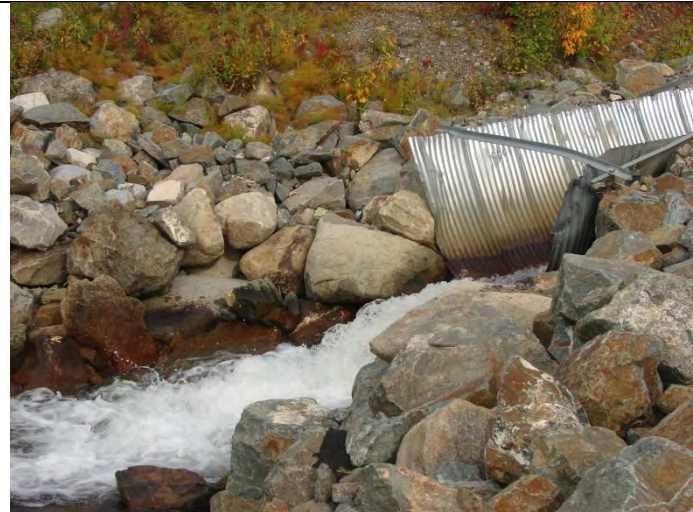
Photograph 6: Close by at the downstream of half-round 2,400 diameter CSP Culvert – 09-10-2013
