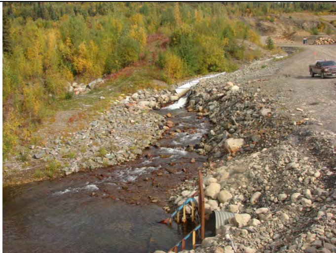
Photograph 7: Looking at half-round 2,400 diameter CSP Culvert discharging to plunge pool – 09-10-2013
