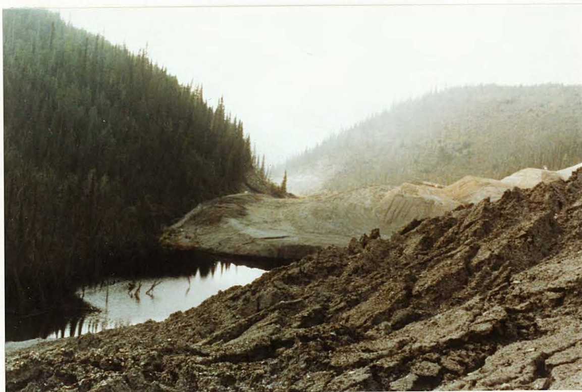
Photo 10: Toe of south tailings lobe. July 1986.
