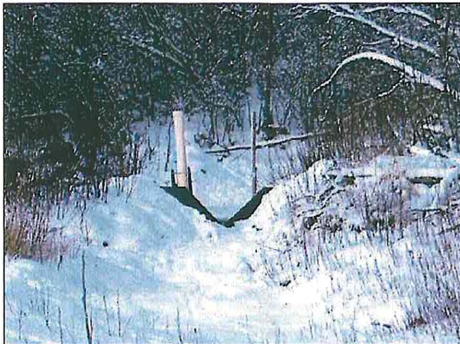
Plate 1 Stilling Well and Staff Gauge Installed Up-Stream of Weir (Looking Upstream)
