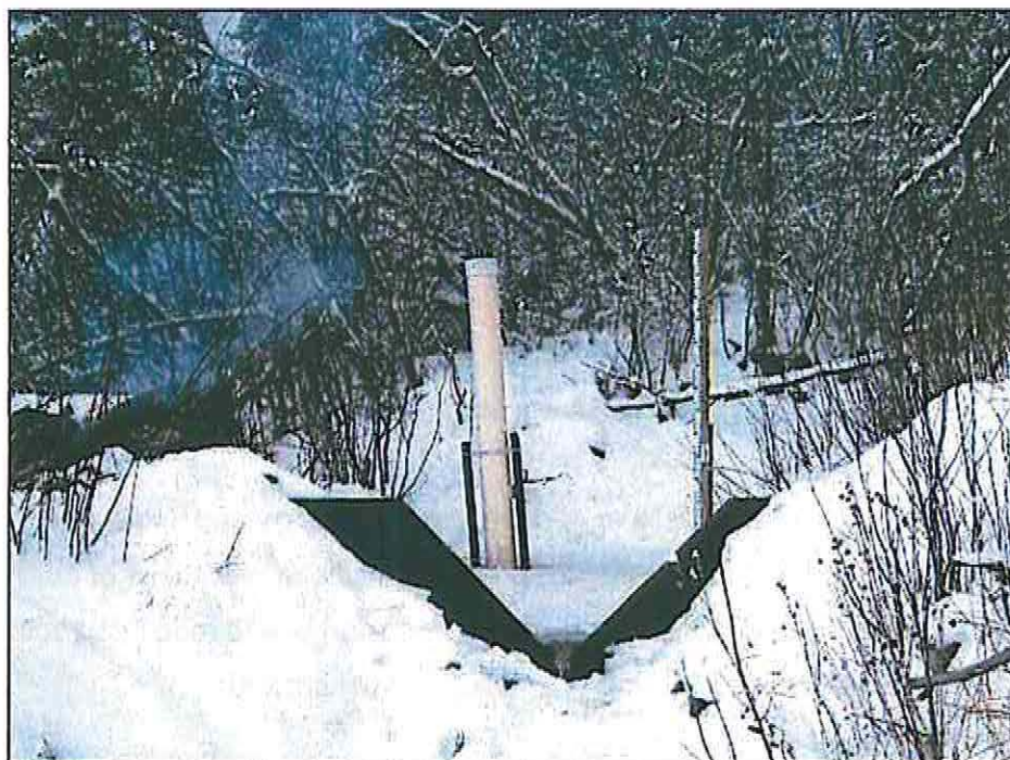
Plate 2 Stilling Well and Staff Gauge Installed Up-Stream of Weir (Looking Upstream)
