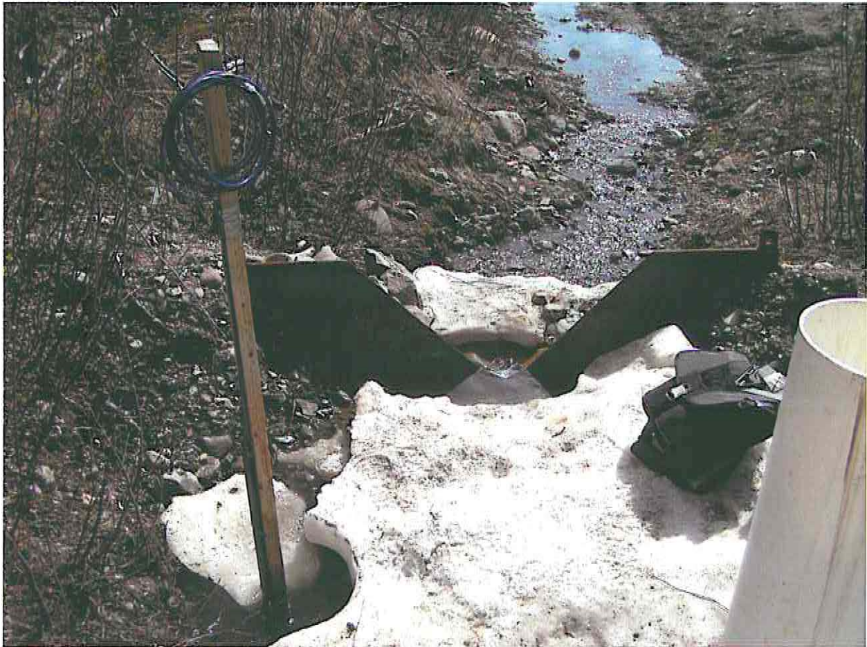
Grum Creek weir looking downstream June 1 2006
