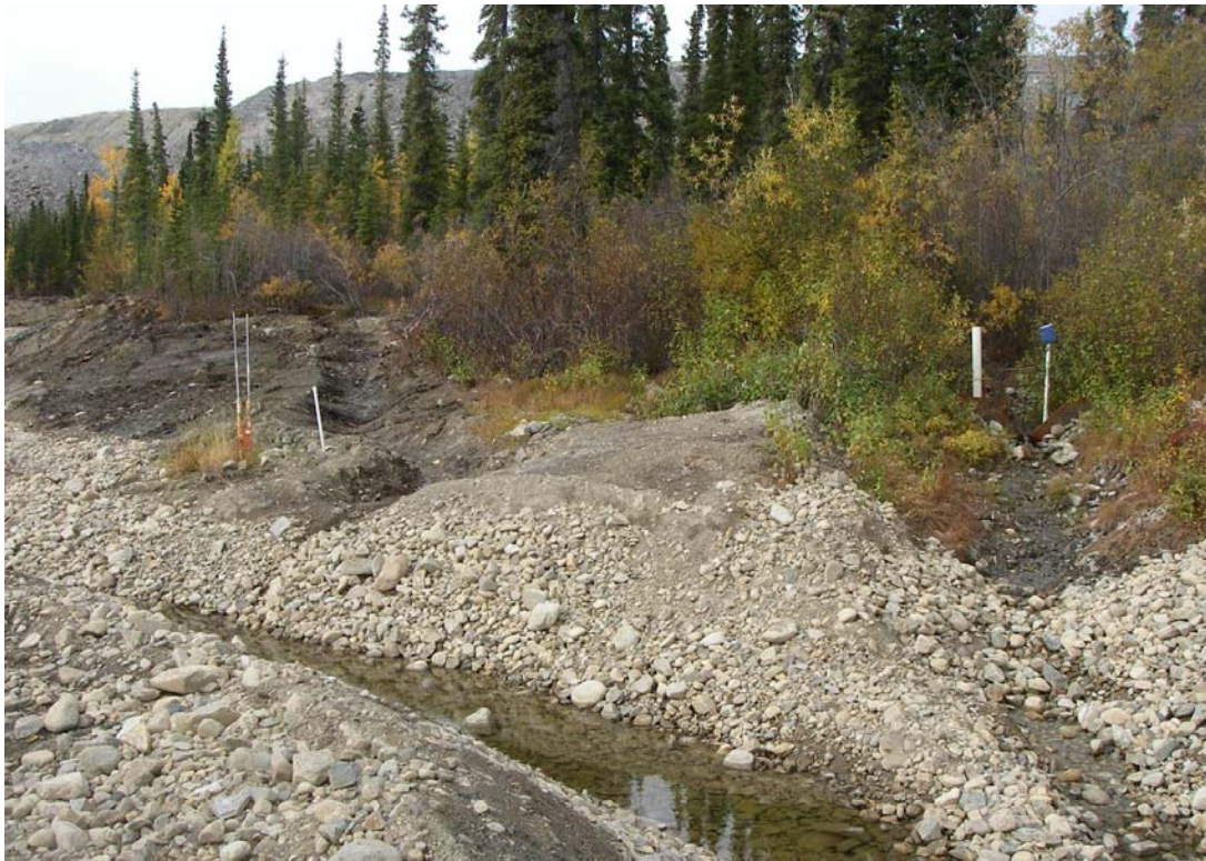
Photo C-6: Seepage flow in V-15 diversion ditch and confluence with Grum Creek.
