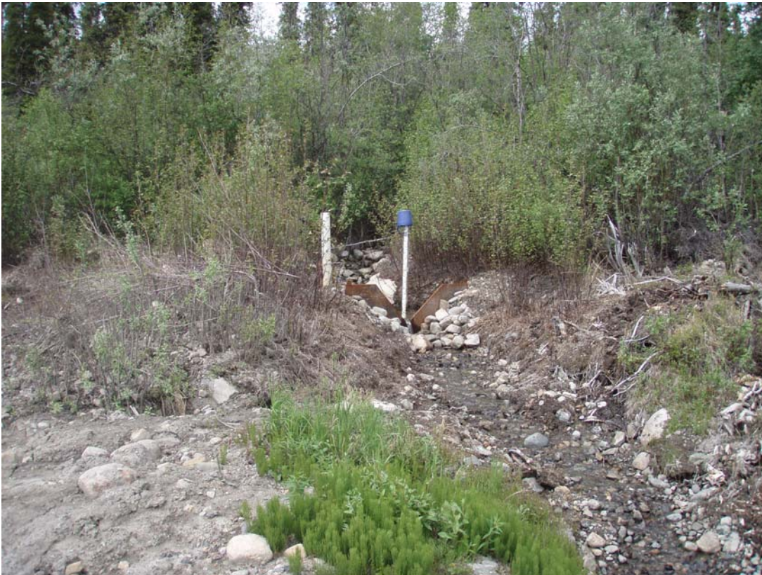
Photo 2: V-notch weir on Grum Creek.
