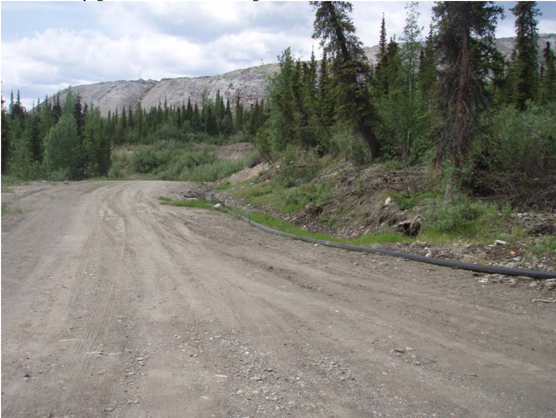
Photo 4: Bank along proposed ditch alignment.
