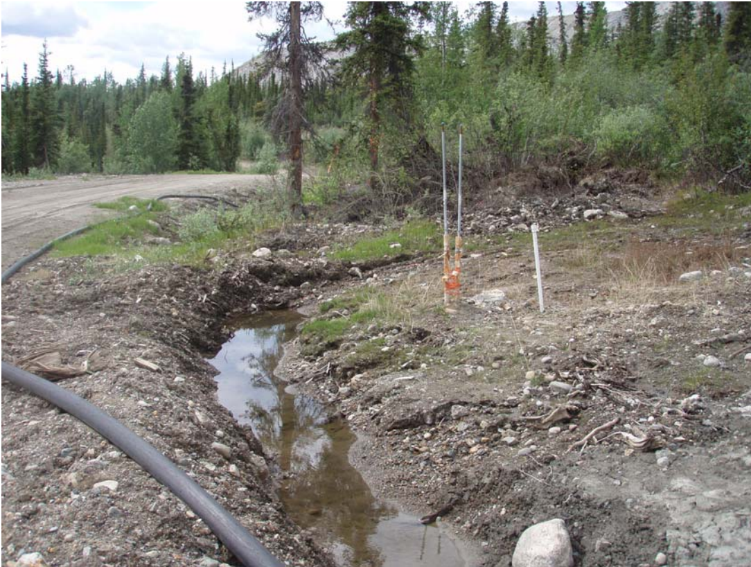
Photo 3: Seepage collection ditch below groundwater wells.
