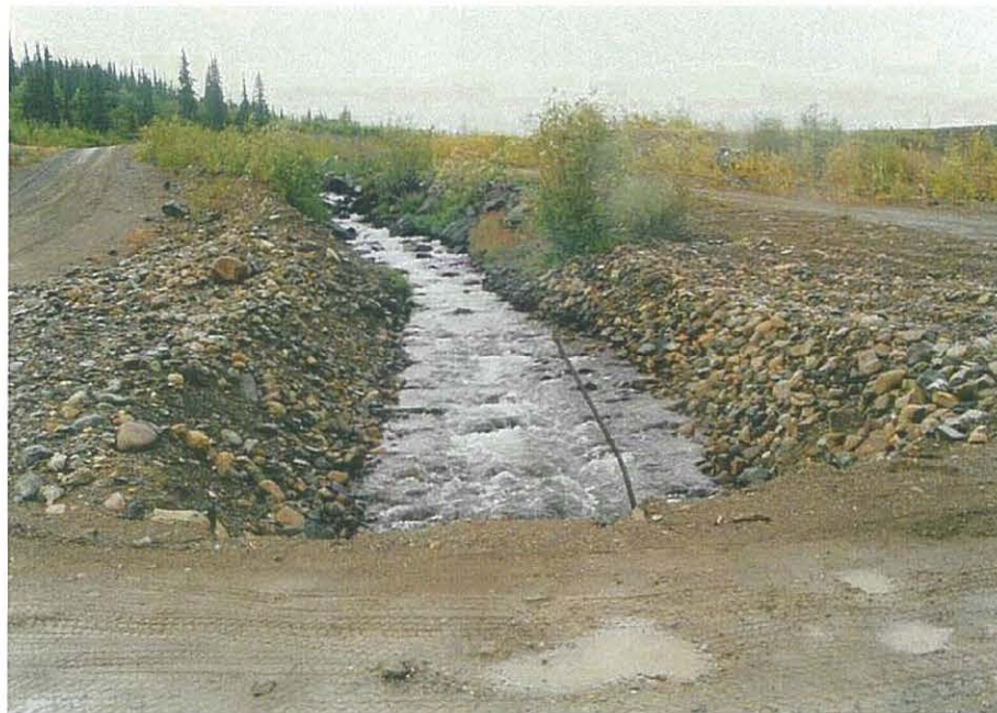
View of the discharge coming down the channel below the Cross Valley Dam.
