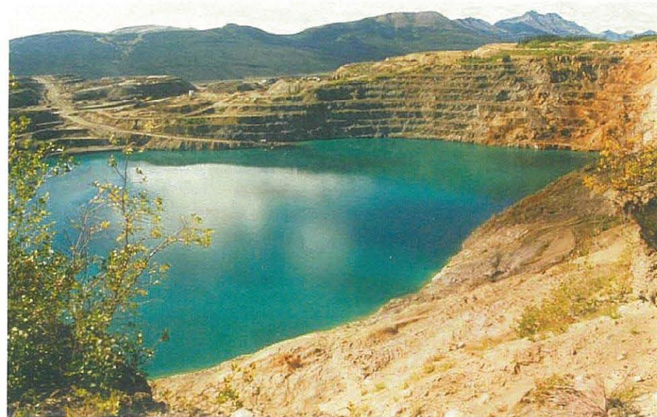
View of Faro Pit. Note failing area in upper right portion of photo.
