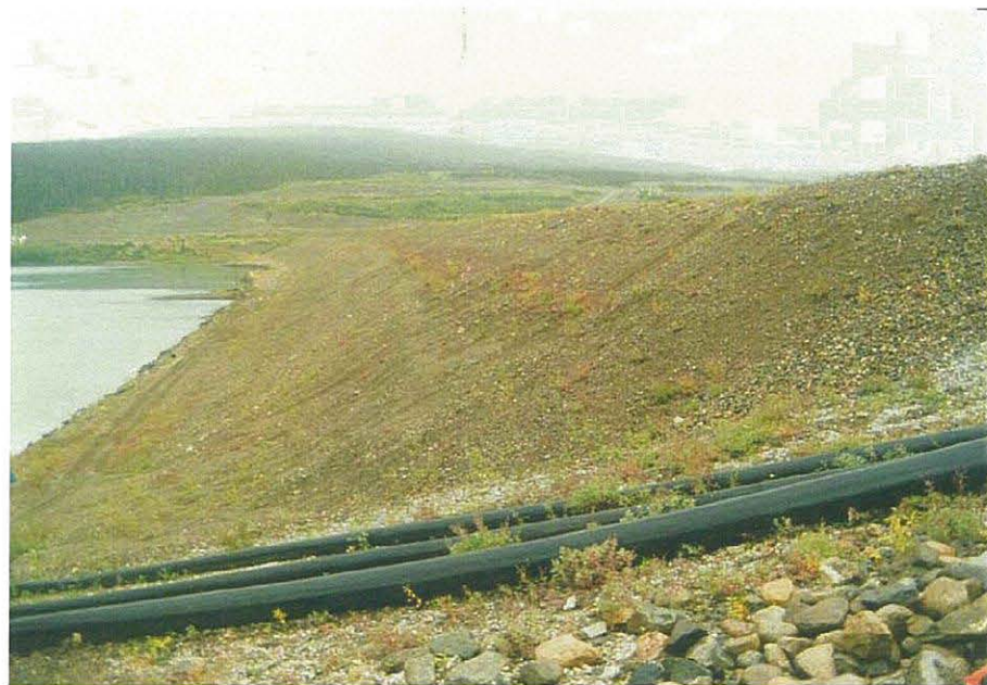
Downstream face of the Intermediate Dam.
