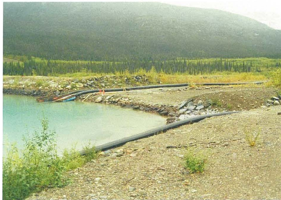
View of entrance to spillway of the Cross Valley Dam.
