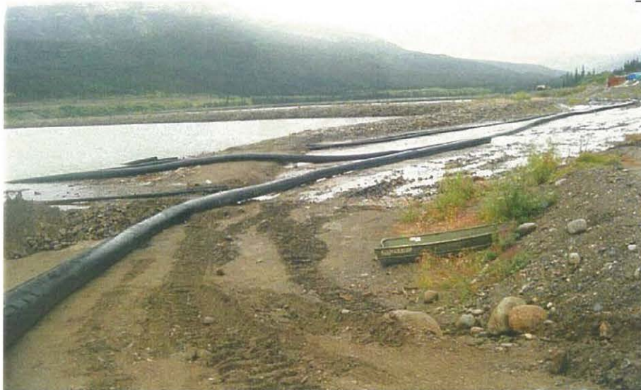
Small berm at entrance of the Intermediate Dam spillway.
