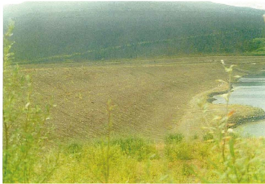
View of downstream face of the Intermediate Dam.
