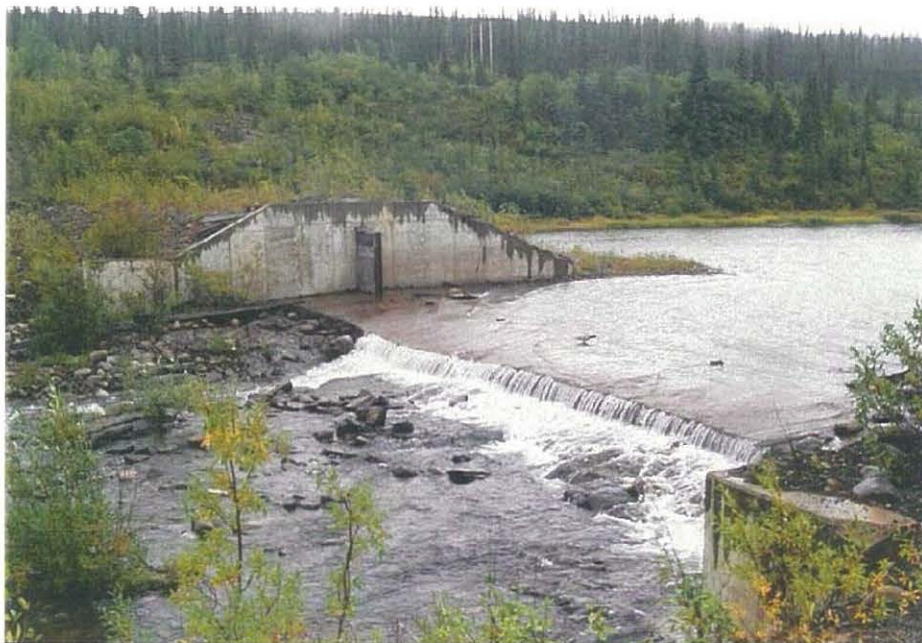
View of the spillway of the FWSD.
