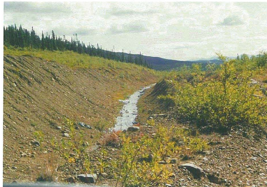
View of the Faro Creek Diversion Channel.
