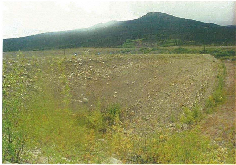
Downstream face of Cross Valley Dam looking towards the south abutment.
