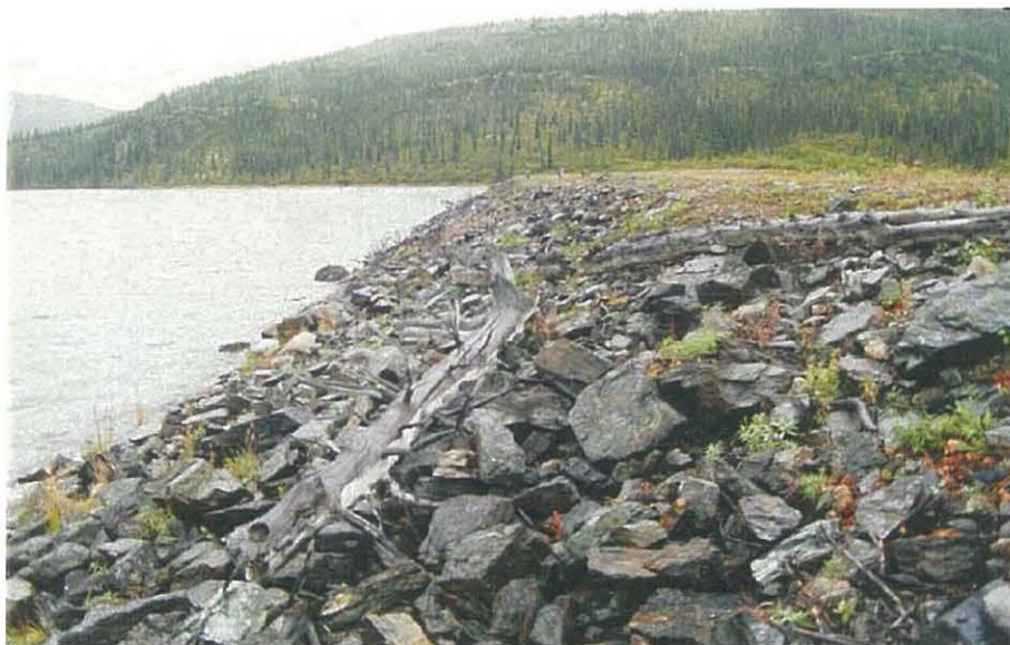
View of the upstream face of the FWSD.
