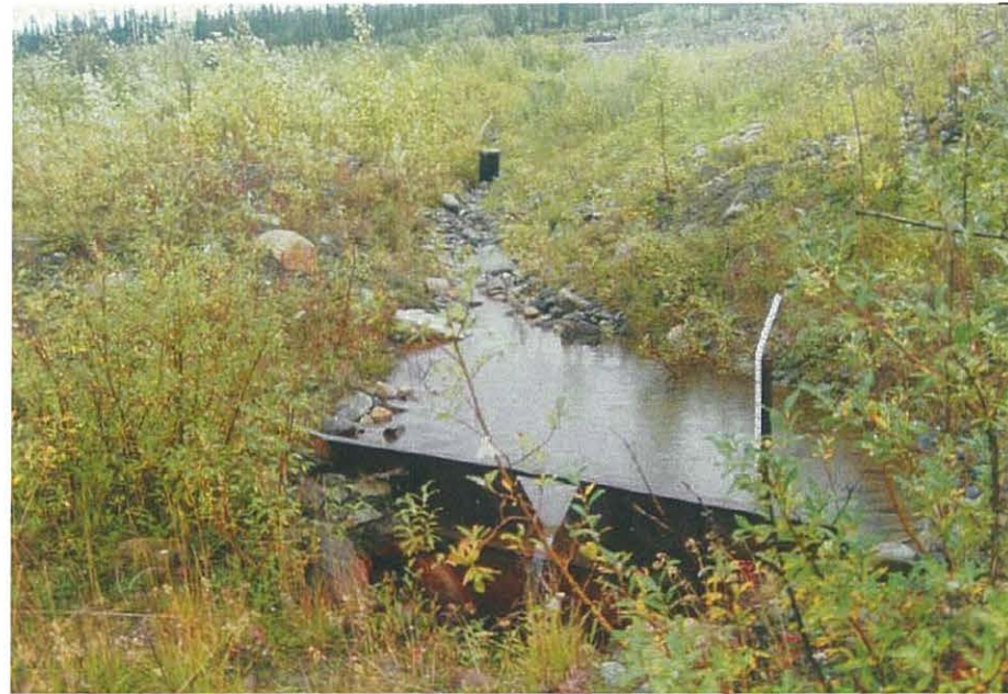
Seepage weir at the toe of the rock-fill berm at the FWSD. Note the location of installation 85-1 in the distance.
