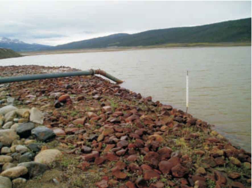
May: Photo shows the pond level at the inlet area to the spillway. and the water level is currently below the staff gauge.
