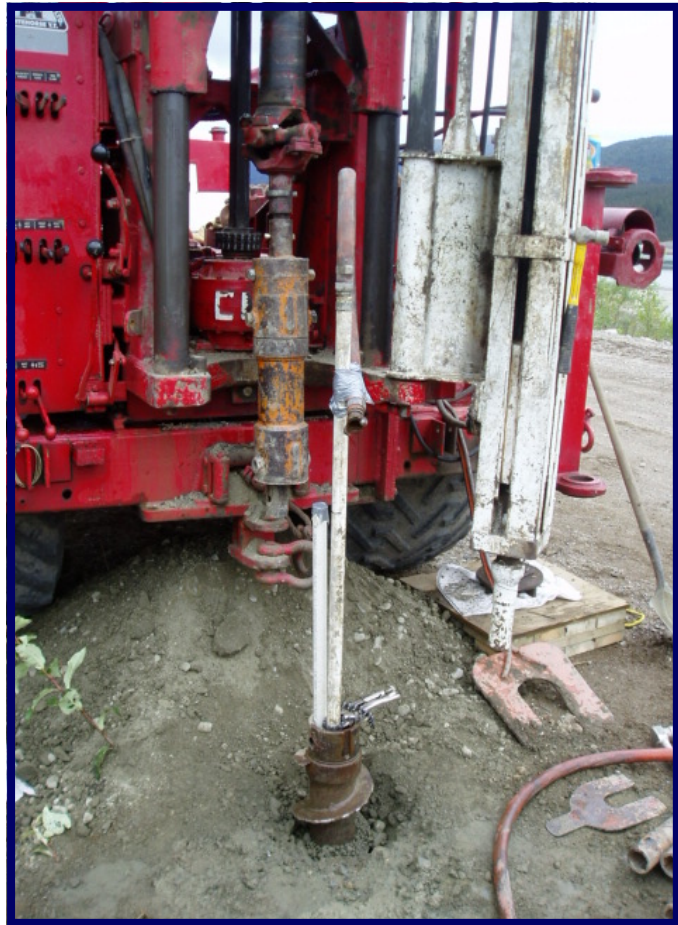
Photo 9 View of a nested pneumatic piezometer installation in BGC05-06.
