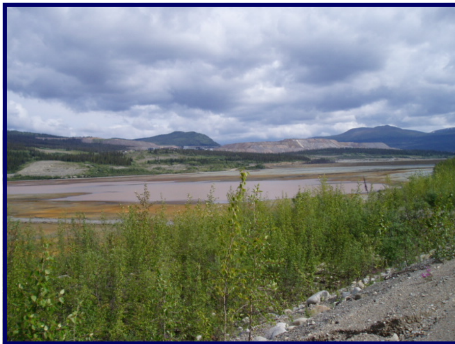
Photo 2 View of Secondary Impoundment Structure, tailings pond and rock dump (in background) from replacement instrument site at BGC05-02.
