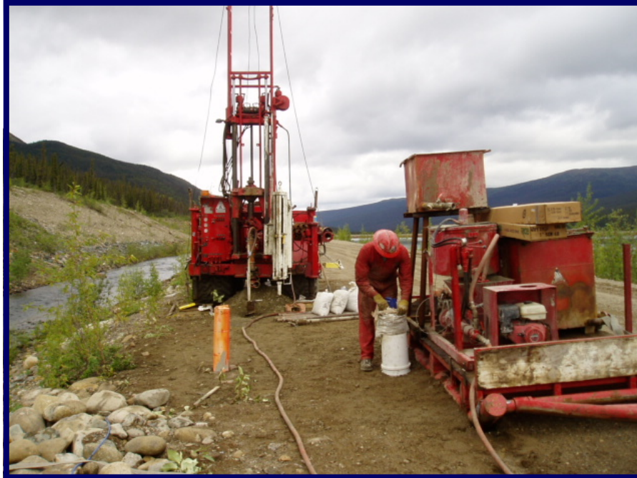
Photo 7 View of drill crew mixing grout for BGC05-03. Note the protective casing around BGC 05-02 in foreground and 1 inch PVC pipe in front of the drill at BGC05-03.
