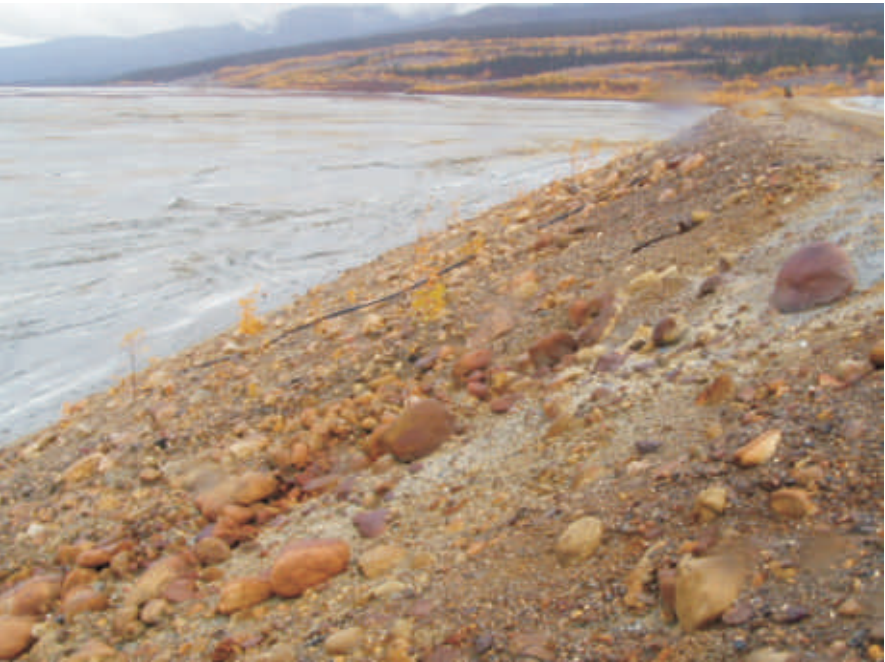
September: Photo shows another view of the downstream side of the face. The face is well armoured with granular gravel, cobbles and boulders. Some vegetation is catching on but in a very sporadic matter. No direct indications of seepage which discharges directly from the face were observed.
