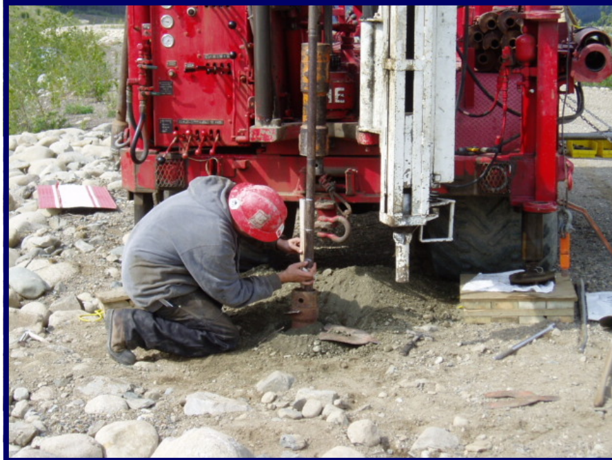
Photo 5 View of drill crew placing 6 inch Standard Penetrometer Test (SPT) marks on drill rod at BGC05-02. Note white SPT hammer to the right of test rod.
