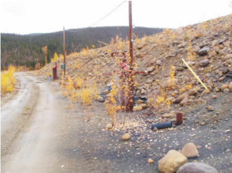
September: Photo shows the downstream face of the far eastern arm overlooking North Fork Rose Creek Diversion. There are cobbles and boulders up to approximately 3 feet in diameter.
