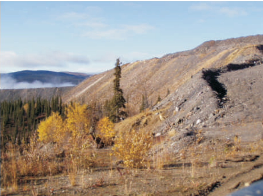
September: view of the face of the waste dumps. No signs of bulging or cracking were noted.
