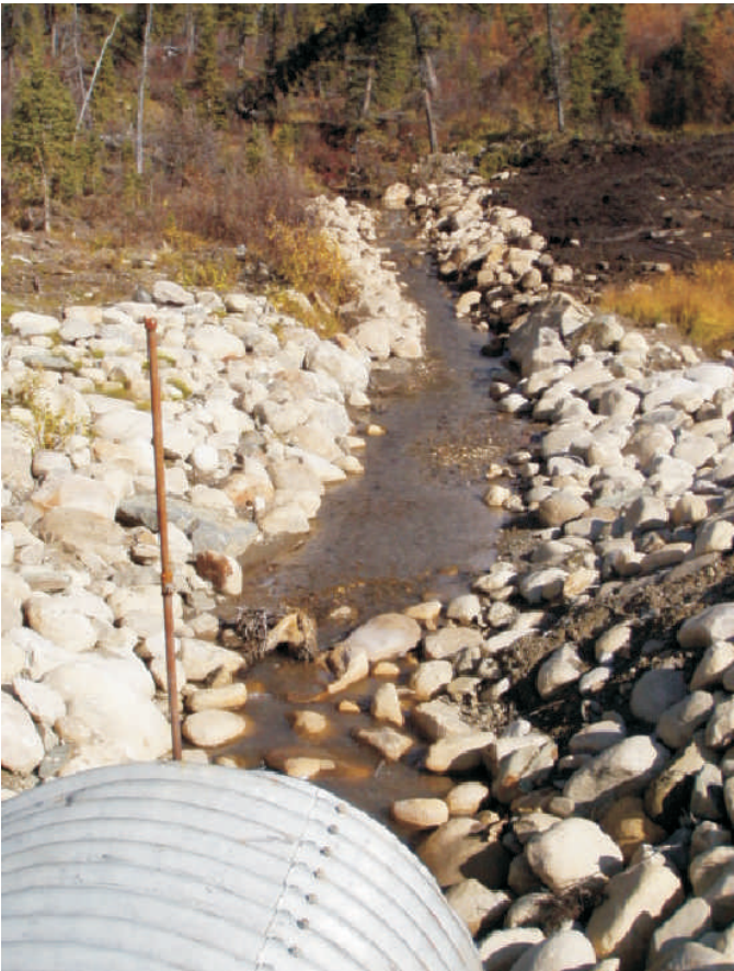
September: Photo shows the channel upstream of the culvert after the construction were undertaken in September.
