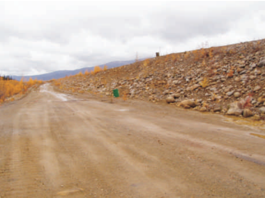
September: Photo shows another view of the downstream face of this dike looking towards the west. Large armouring from the cobbles and boulders is located on the face.
