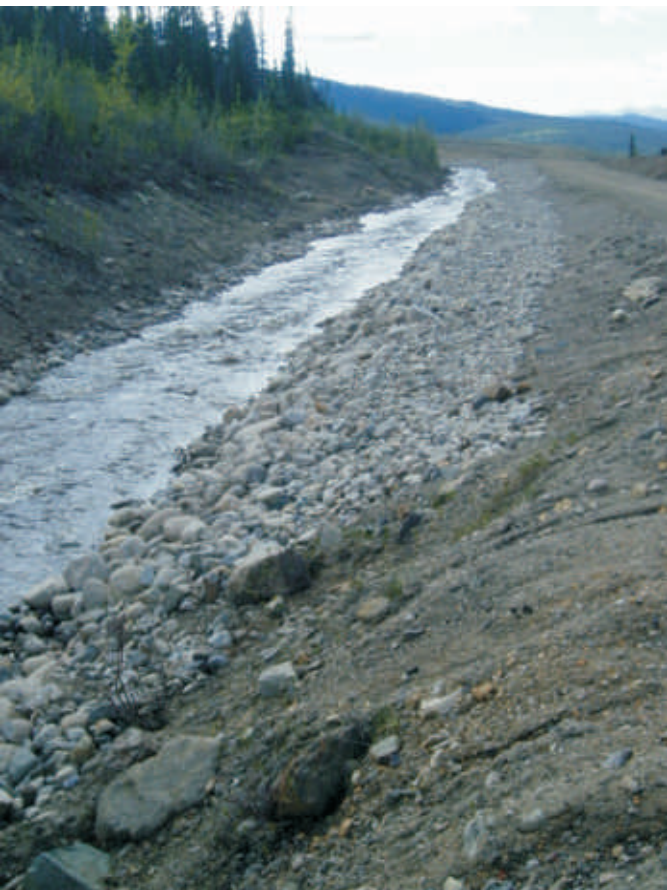
May: Photo shows the beginning of the next section of the pilot channel. This is located some approximately 100 metres downstream from the corner.
