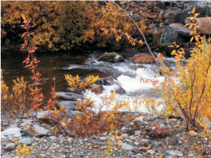
Photo shows a view of the water flowing over top of the first weir. The central boulders have been pushed out of the way but the weir is still effective in discharging energy.
