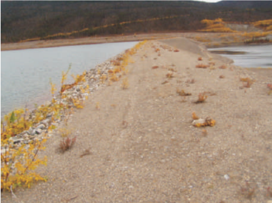
September: Photo shows a view of the crest looking towards the south. The crest appears to be properly graded with no signs of settlement or standing water.
