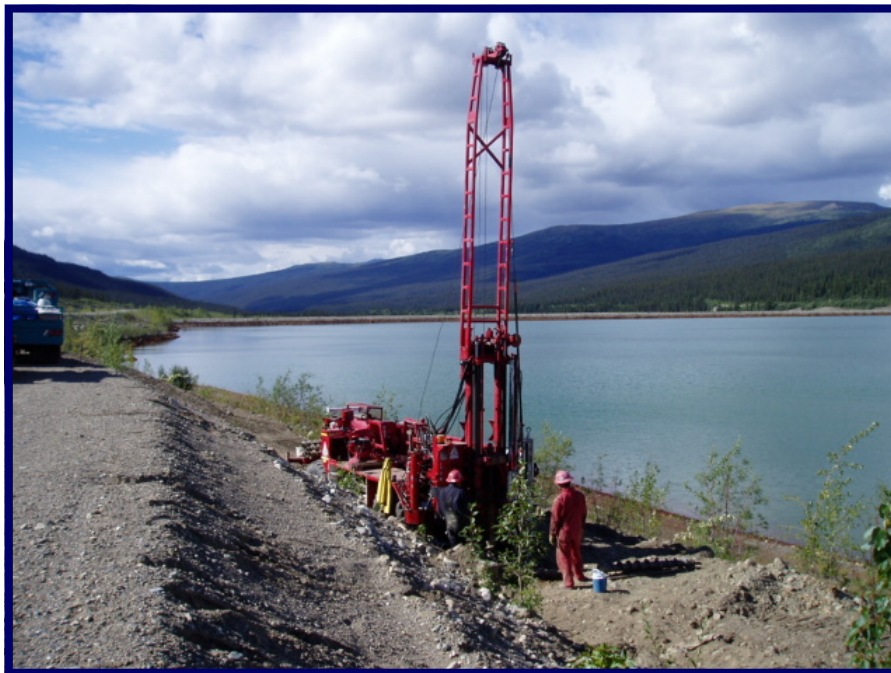
Photo 8 View of drill and crew at instrument replacement location at BGC05-06 with Intermediate Dam and pond in background.
