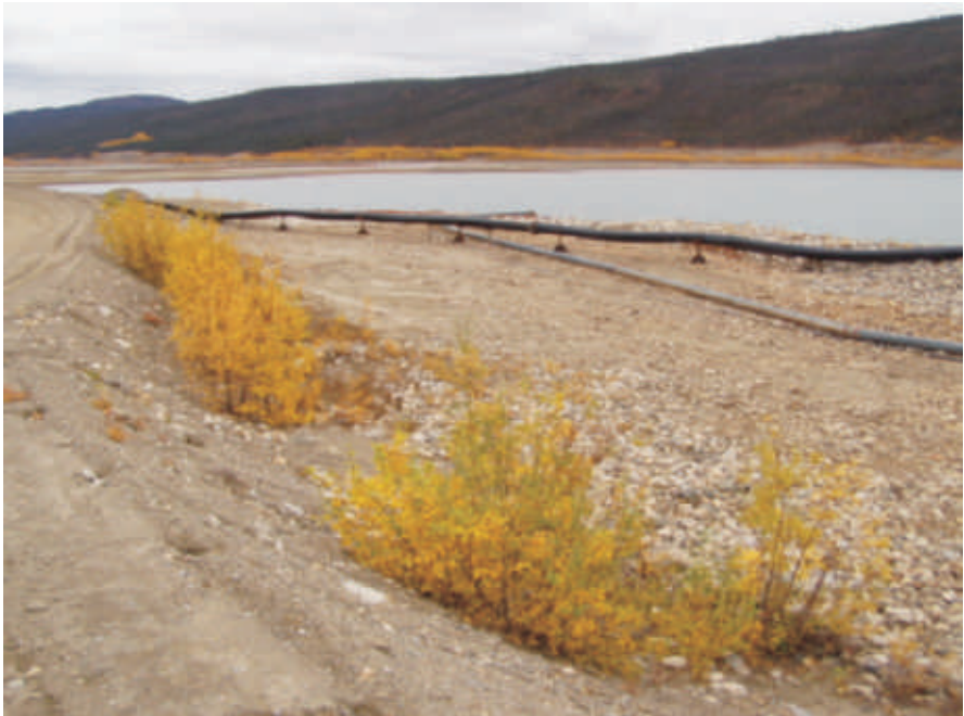
September: Photo shows the current condition of the inlet to the spillway. No water is currently flowing in the spillway.
