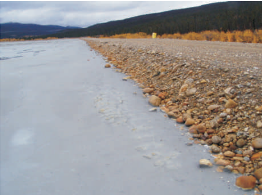
September: Photo shows the upstream side of this crest. Approximately 0.8 m to 1 m of freeboard exists from the tailings surface to the crest of the dam.
