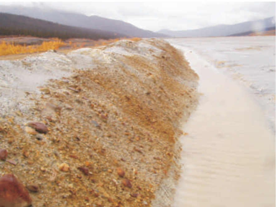
September: Photo shows a ditch on the upstream side of the Secondary Dam. There is approximately 1.2 to 1.5 m of freeboard from the ditch water level to the crest of the dike.
