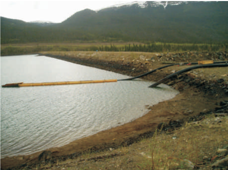
May: Photo shows the inlet into the spillway on the Cross Valley Dam and also the two siphon pipes.
