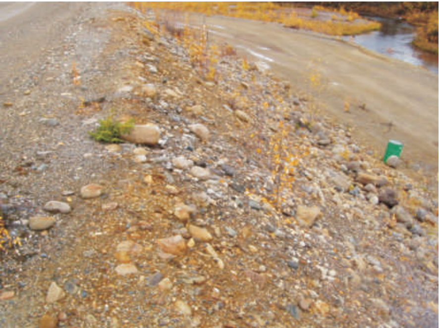
September: Photo shows the downstream face which is heavily armoured with gravel, cobbles and boulders.
