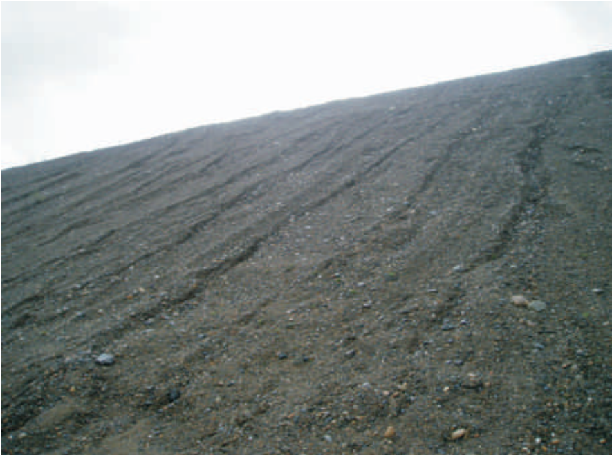
May: Photo shows a number of different sized erosional gullies on the downstream face.
