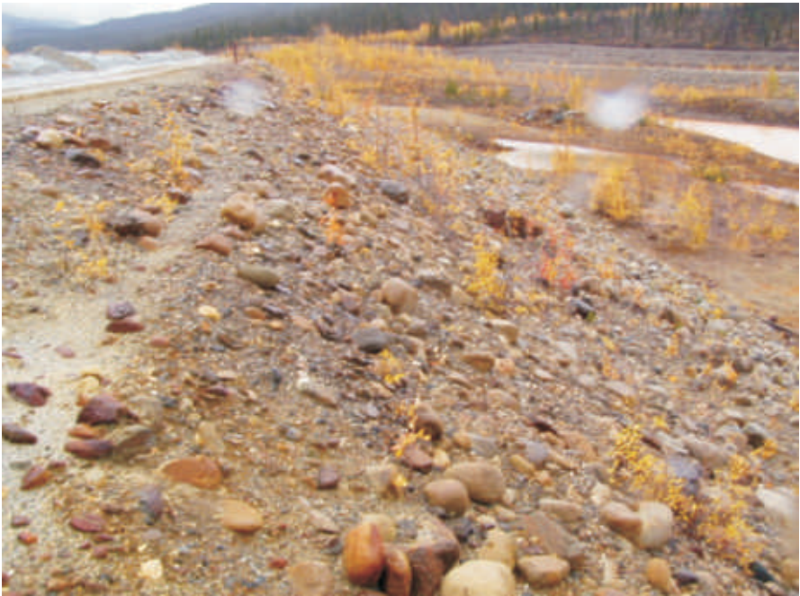
September: Photo shows a view of the downstream face of this dam. There is the occasional erosional gully but the coarse material appears to prevent any erosion of the face.
