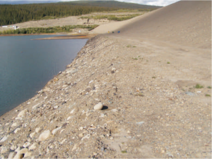
August: Photo shows a view looking along the edge of the Polishing Pond.
