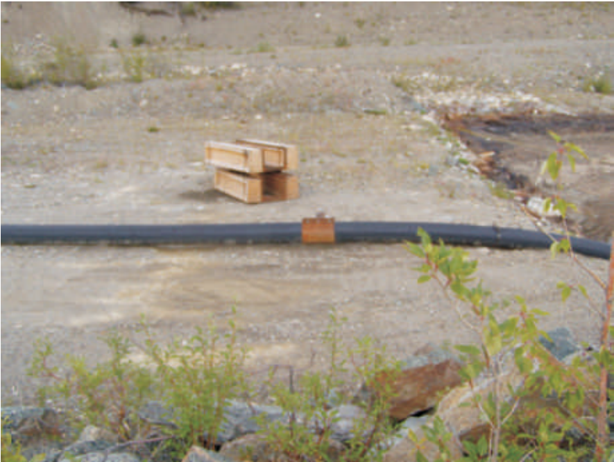
August: Photo shows a view of the Emergency Spillway on the Cross Valley Dam.
