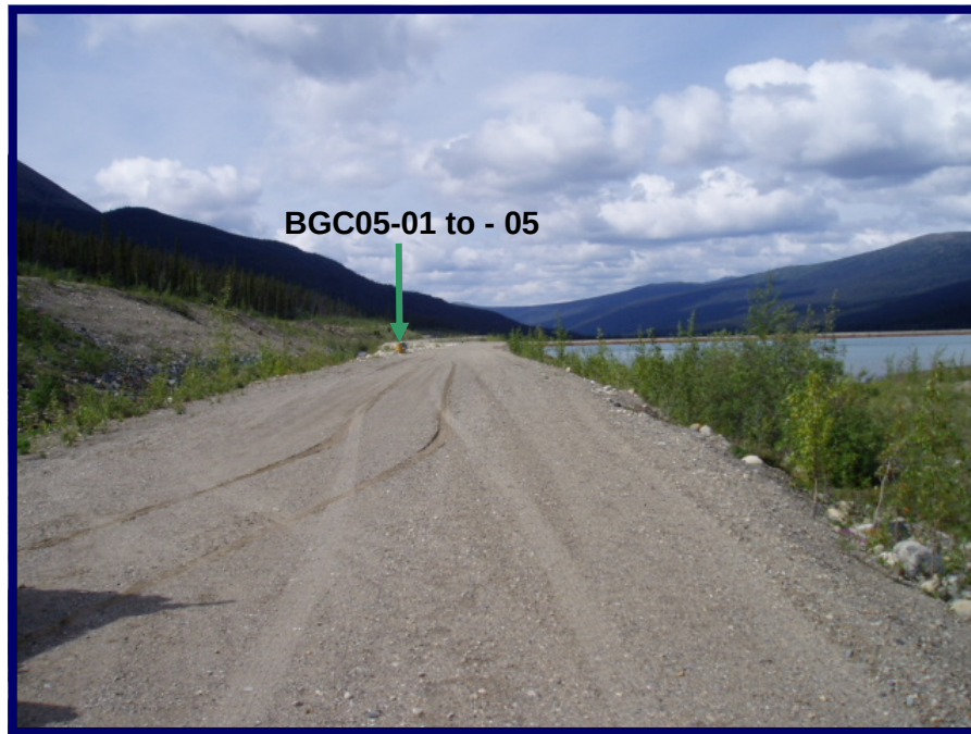
Photo 1 View of Rose Creek Diversion Canal Dike looking west along the crest. Note the barrels on left side of photo indicating location of replacement instruments.
