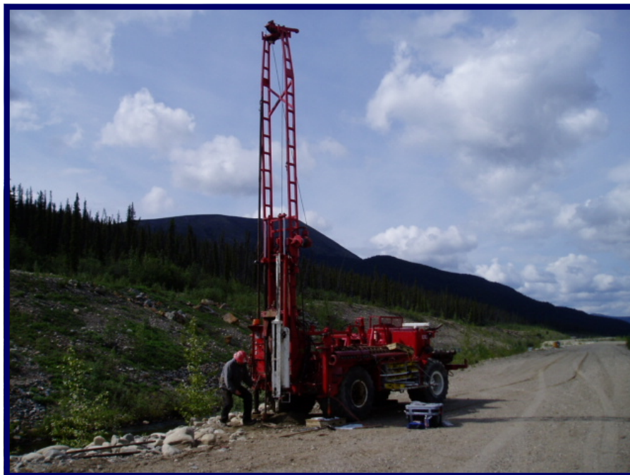
Photo 4 View of drill and crew at instrument replacement location at BGC05-02.
