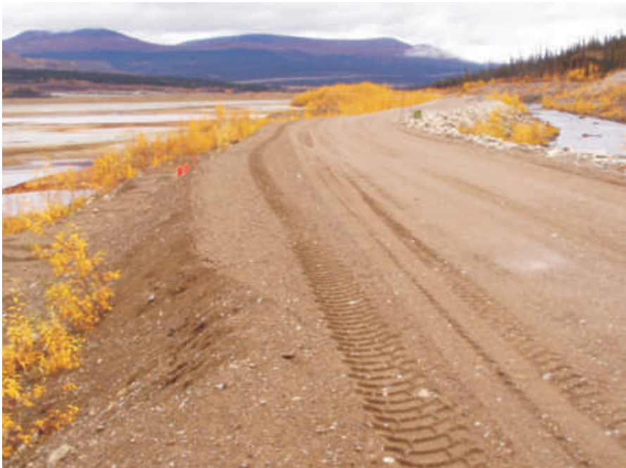
Photo shows a view of the regraded crest located at approximately CD-21. On the left can be seen 3 new instrumentation casings.
