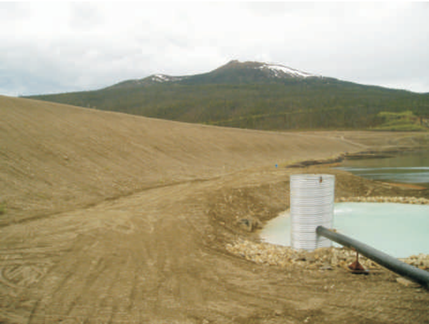
May: Photo shows another view of the downstream side of this dam. No signs of seepage, discharge or standing water were noted on the toe.
