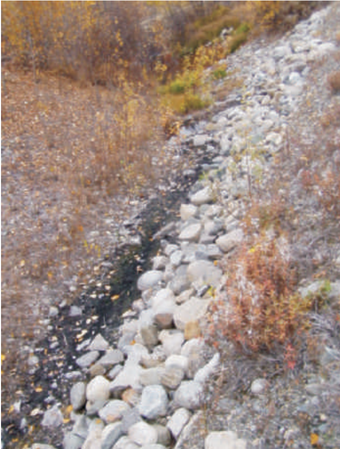
September: Photo shows the bottom of the seepage collection trench looking north towards the middle V-Notch Weir. As can be seen the bottom of the trench is relatively dry, possibly a result of the ongoing pump test.
