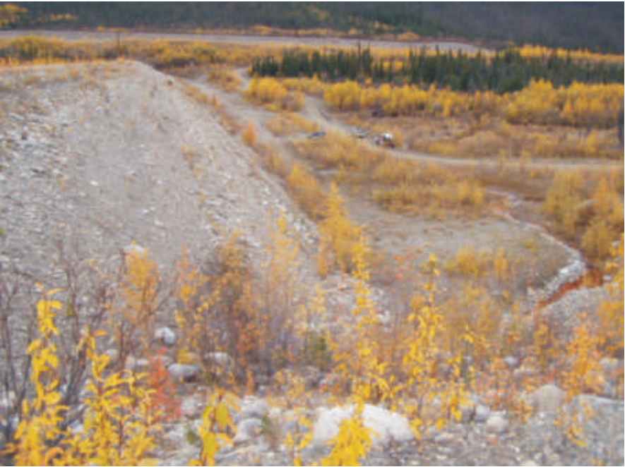
September: Photo shows a view of the downstream face and toe area where the pump test is ongoing. The seepage collection trench appears to be slightly drier than typical, likely in relation to the ongoing large scale pump test.
