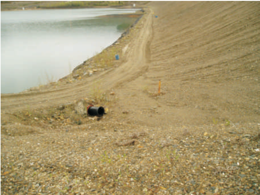
May: Photo shows the toe at the south abutment. As can be seen, there are no signs of seepage discharging in this area, where seepage has been noted in previous years.
