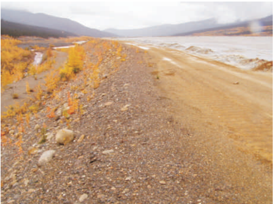
September: Photo shows the crest looking west towards the Intermediate Dam. This dam is constructed out of sand and gravel with armour on the downstream side consisting of large rounded cobbles and boulders. On the upstream side, tailings come close to the upstream crest of the dam.
