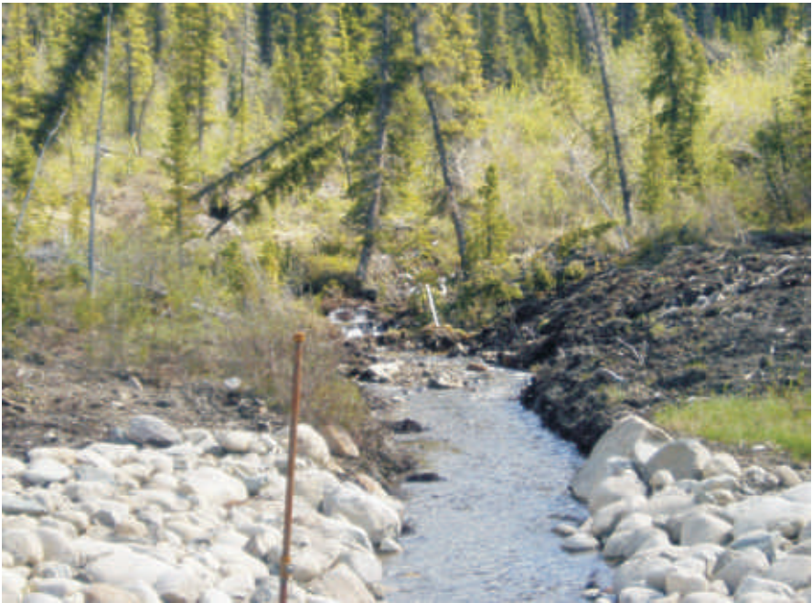
May: Photo shows the outfall section of the NVWID.
