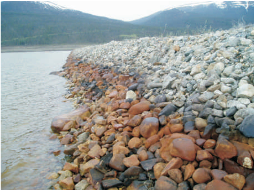
May: Photo shows the riprap on the upstream side.
