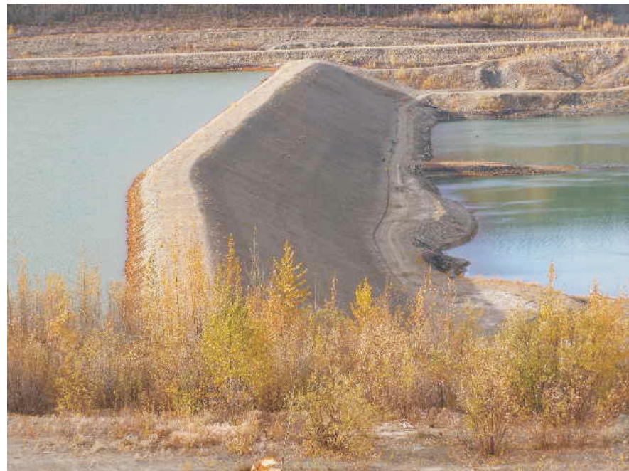
September: shows the downstream slope and crest of the Intermediate Dam.
