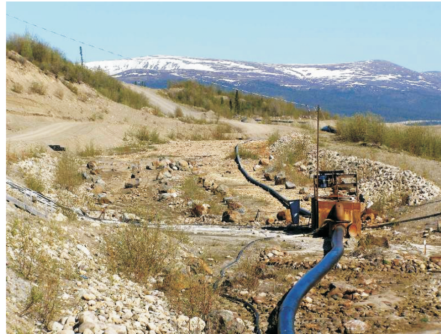
June: Middle portion of spillway, including large boulders.
