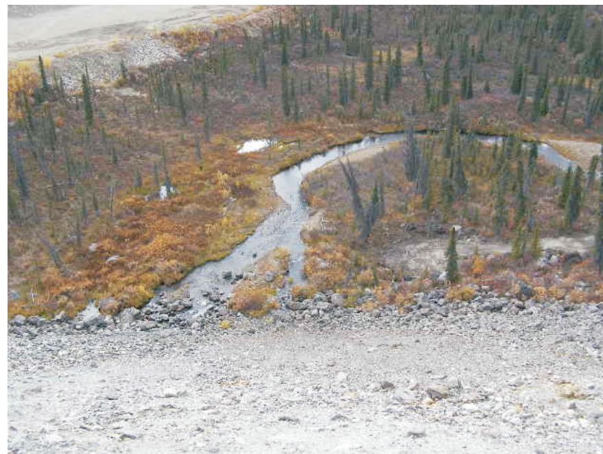
September: shows the discharge emerging from the bottom of the rock drain. The creek configuration appears consistent with previous years. There are no signs of sloughing or ongoing problems with stability.
