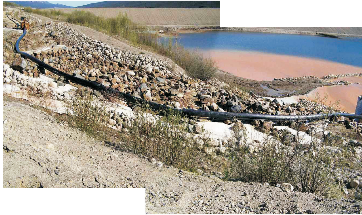
June: Two shot panorama showing the lower steep section of the Intermediate Dam Spillway. Note the riffle/pool form of this section of the spillway.
