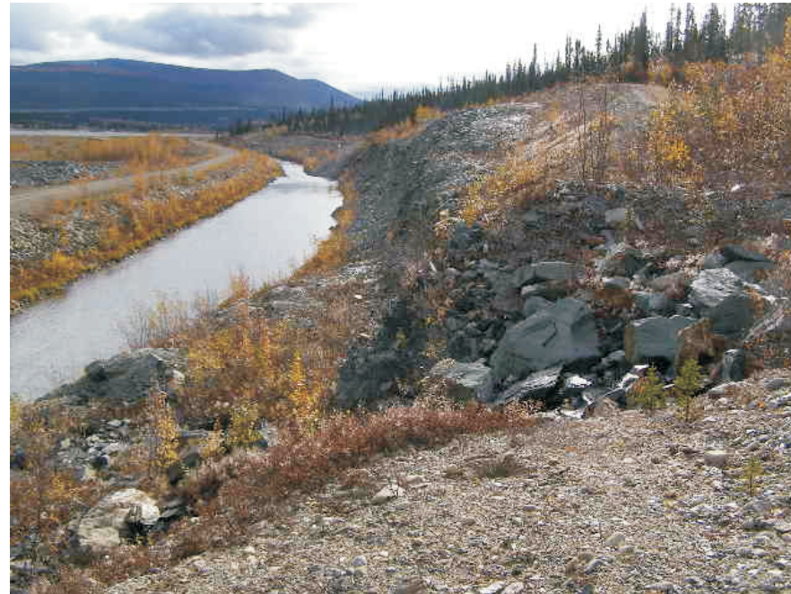
September: looking in the upstream direction at the canal and the backslope.
