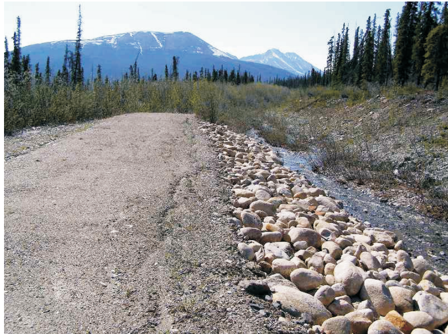
June: The deflection berm area near the guard house.
