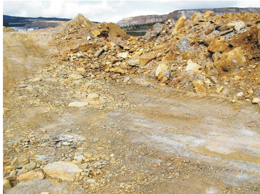
June: shows a view looking upslope towards the main part of the breach in the dam. Note, in the foreground, the appearance of tailings.
