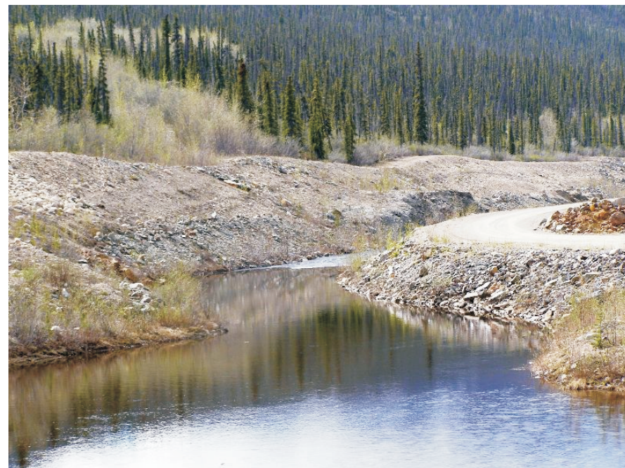
June: looking in a downstream direction at the location of the 1981 Diversion Dam.
