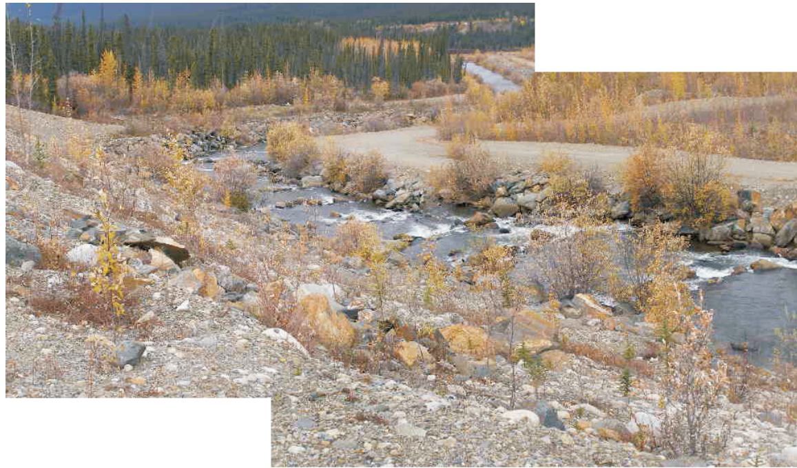
September: panoramic view showing the condition of the weirs located within the upper weir section. A number of the central boulders have been displaced due to concentrated water flow.
