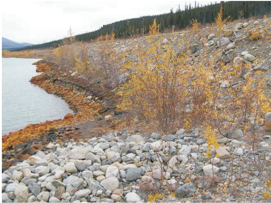
September: lower edge of the Rose Creek Diversion Canal/spoil pile adjacent to the Intermediate Pond.
