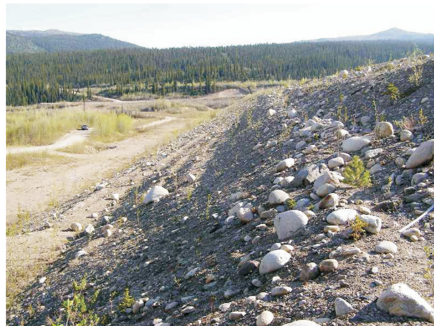
June: View along downstream face of the dam.
