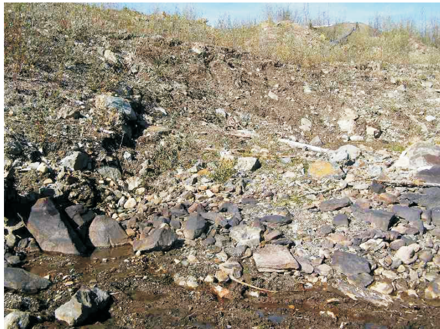
June: Headscarp formed near seepage discharge.
