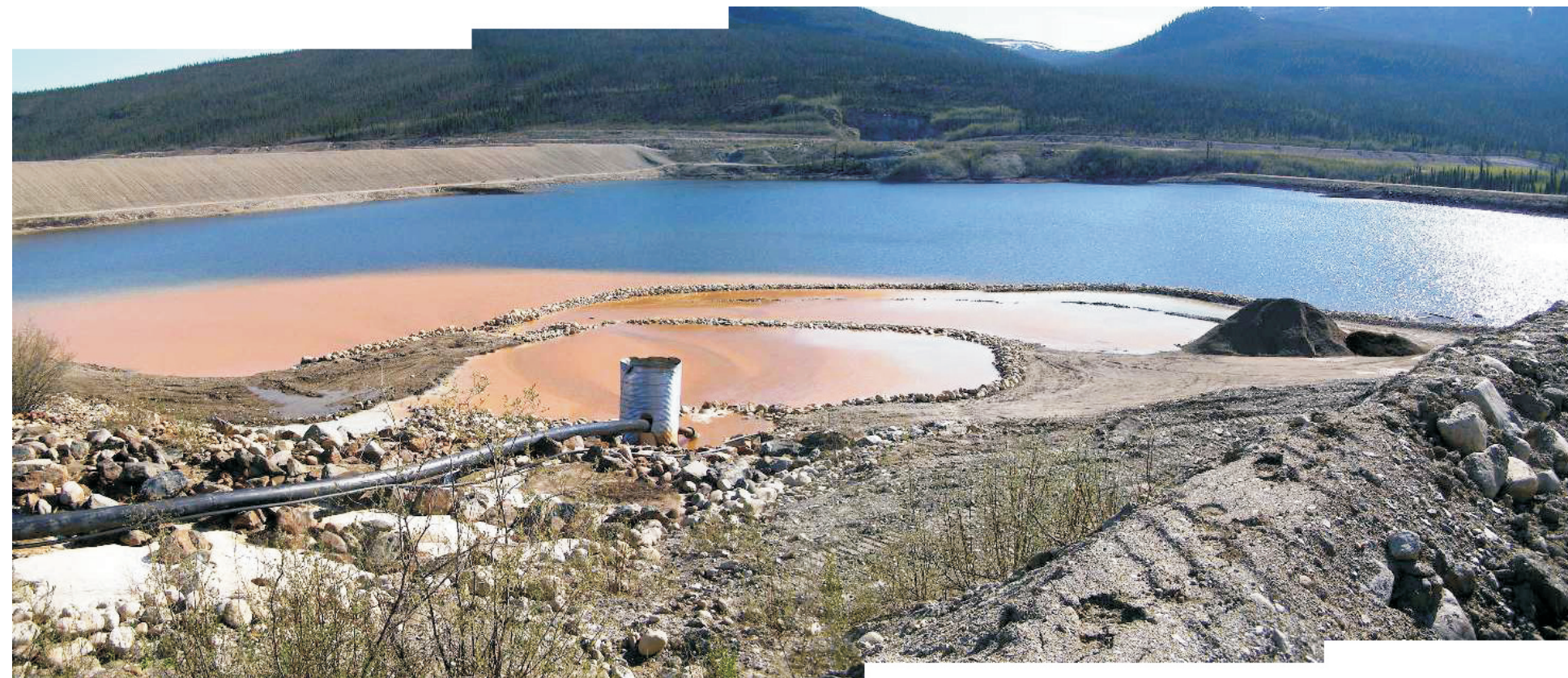
June: Three shot panorama showing the sludge collection area built at outlet of the Intermediate Dam Spillway.
