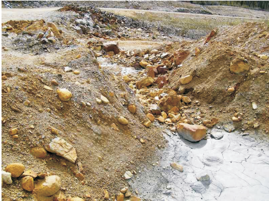
June: shows a view of this breach in the Secondary Tailings Dam. The tailings were washed into the Intermediate Impoundment.
