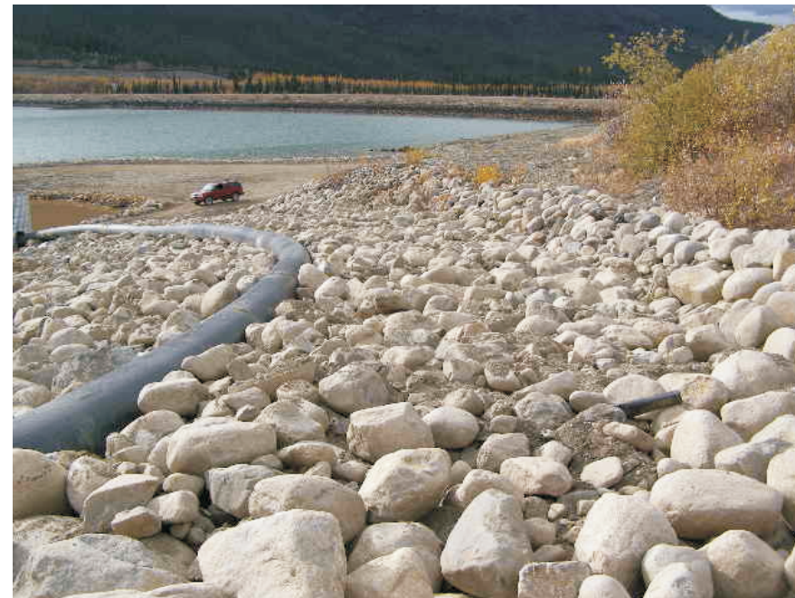
September: another view of the recently repaired riprap.
