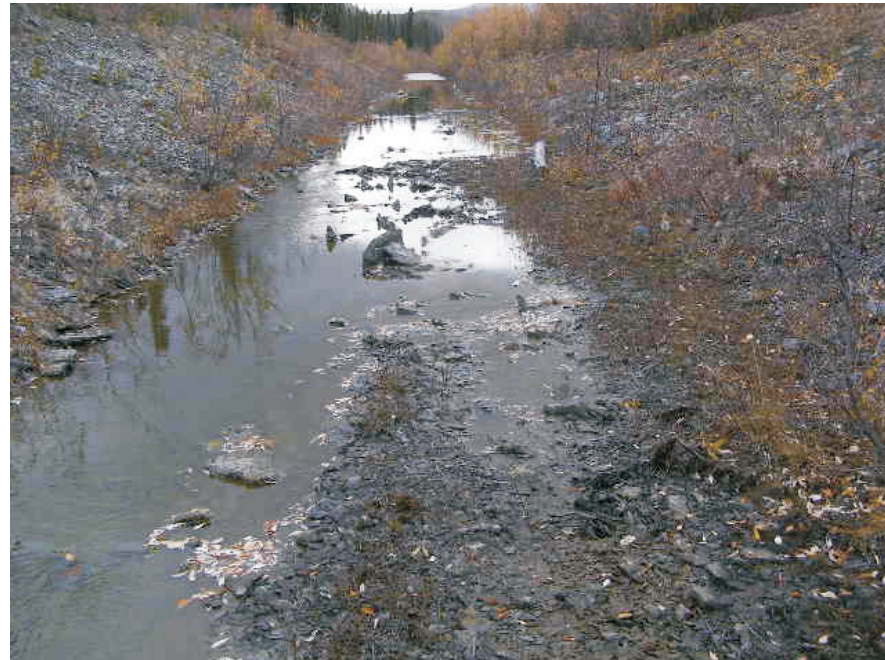
September: is a view of the ditch bottom looking in an upstream direction.
