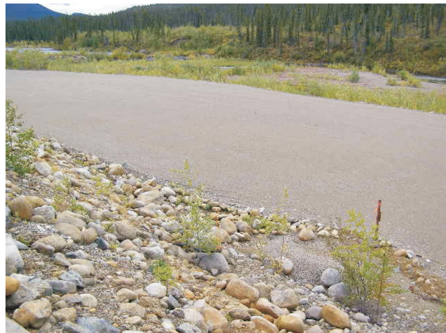
August: lower road surface near pumphouse pond, showing the re-graded surface.
