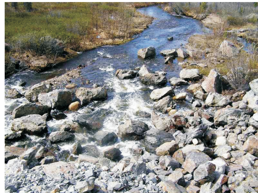
June: shows a view looking at the creek as it flowing out of the base of the Rock Drain free and clear with no obstructions.
