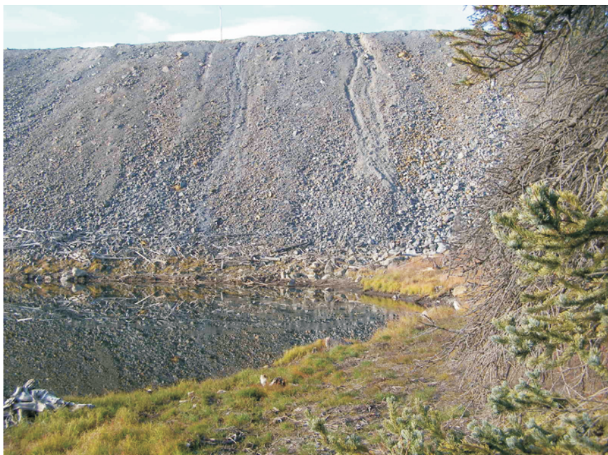
September: view of the upstream side of the North Fork Rock Drain. Note that some of the driftwood below the water line has been removed.
