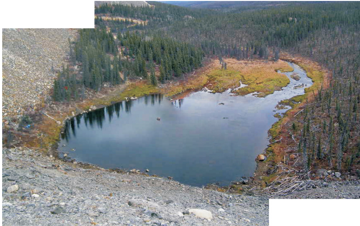
September: a panoramic showing the head pond on the upstream side of the North Fork Rock Drain. The pond appears slightly lower than last year at this time. From this perspective, there does not appear to be any signs of significant sloughing or erosion ongoing.
