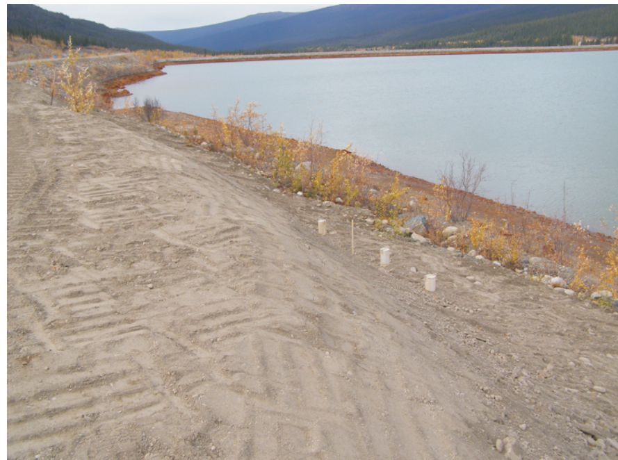
September: same location as in the photo above. Note that the oversteepened slope has been backfilled.
