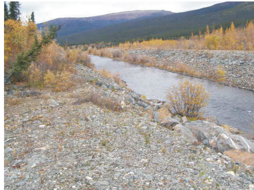
September: shows a view looking downstream on the canal. As can be seen, this is a low gradient part of the diversion between the upper and lower weir sections.
