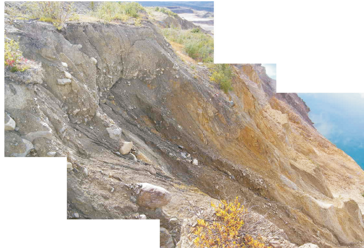
September: Three shot panoramic of seepage discharge area in Faro Pit wall.
