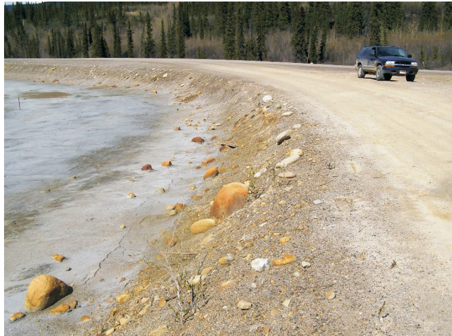
June: shows a view of the abutment of the Secondary Tailings Impoundment as it meets the main road.
