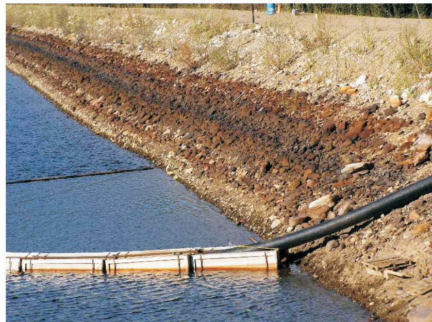
June: Water level is below the lowest elevation of the riprap protection.
