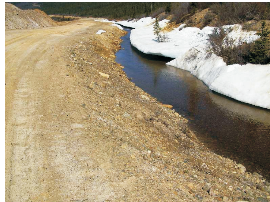
June: Northern leg of the diversion. Note the overhanging banks of snow and ice.
