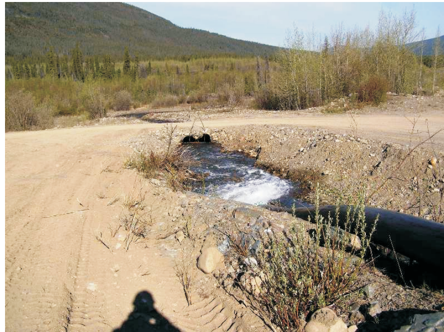
June: Siphon discharge at lower end of spillway.
