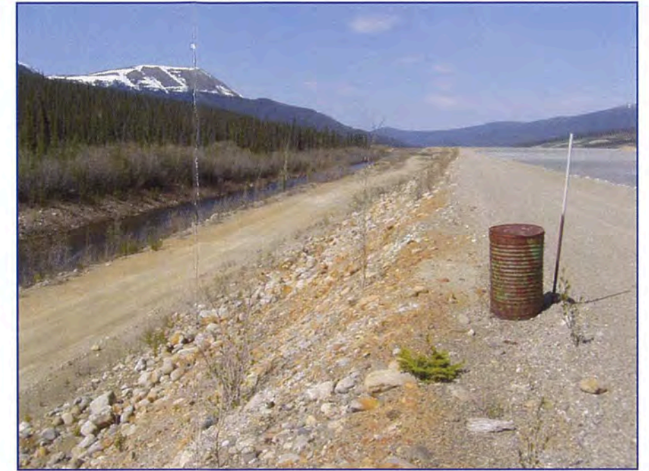
June: a view of the downstream face of the dam with the diversion channel on the left side of the photo.
