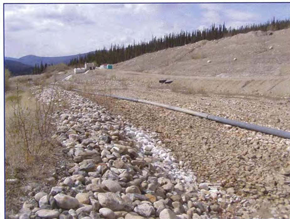
May: looking downstream in the dam spillway.
