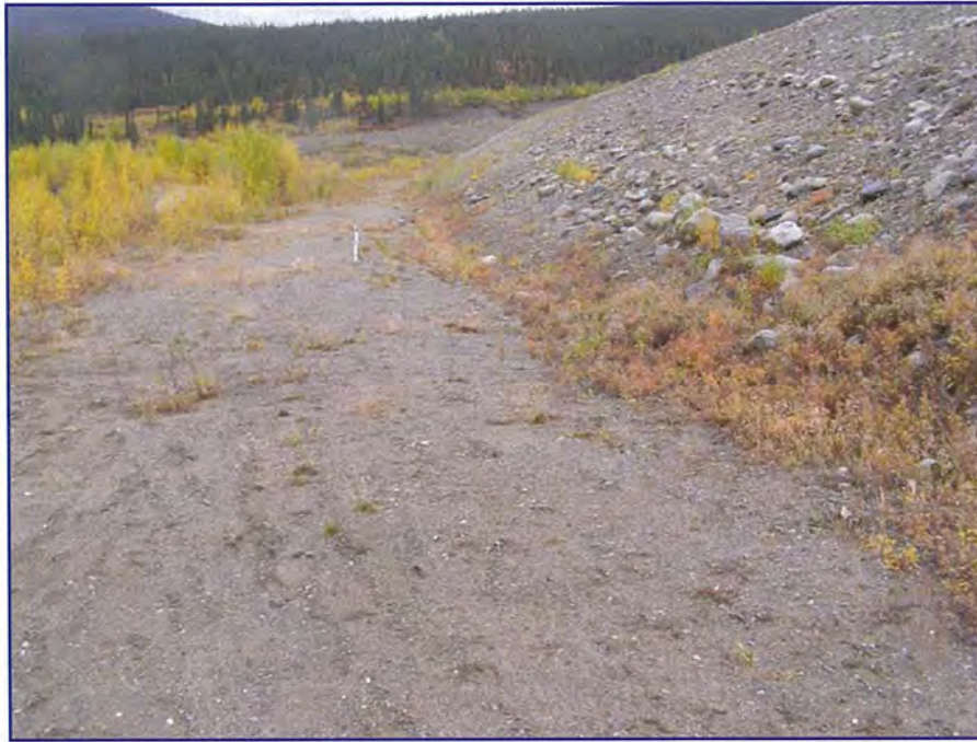
September: shows a view of the downstream toe, some vegetation remains after the 2007 removal, but is low priority to be removed.
