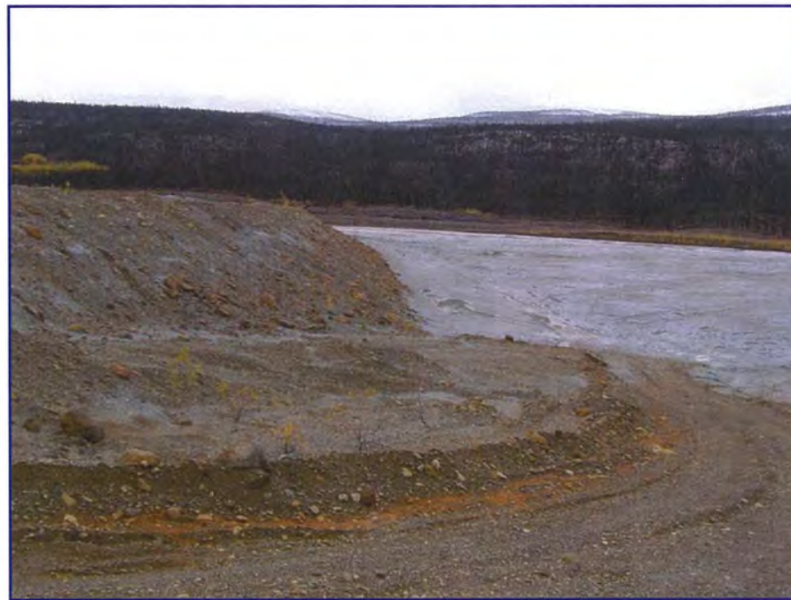
September: shows the downstream face of the Secondary Dam.
