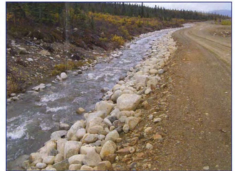
September: shows a view of Faro Creek Diversion looking upstream.
