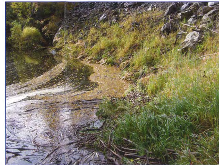
September: a view of the sediment and grass that is present on the upstream face of the rock drain.
