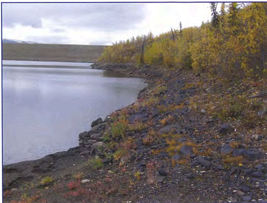
September: a view of the toe of the spoil pile. There were 25 seepage discharge locations. The pond level is 1.9 m lower than usual.
