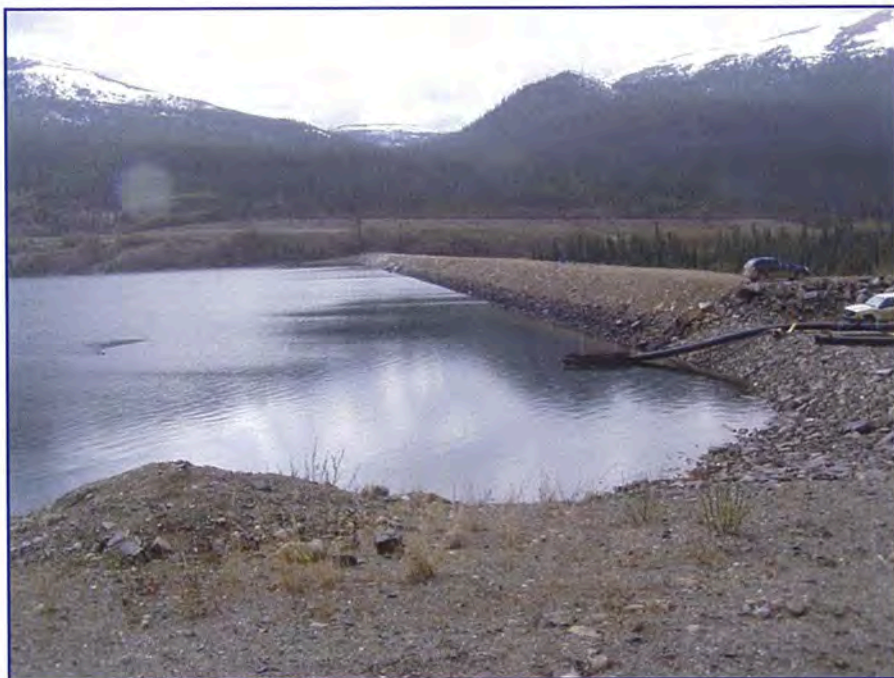
May: shows the upstream face of the Cross Valley Dam
