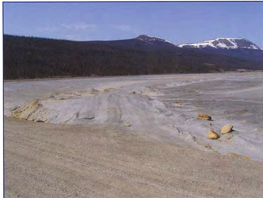
June: shows a view of the Primary tailings dam crest.
