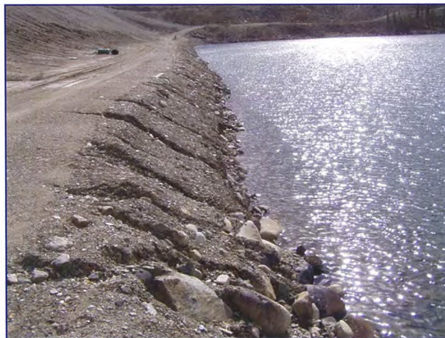
May: shows a view of the edge of the polishing pond. Note that some rilling and wave erosion is evident.
