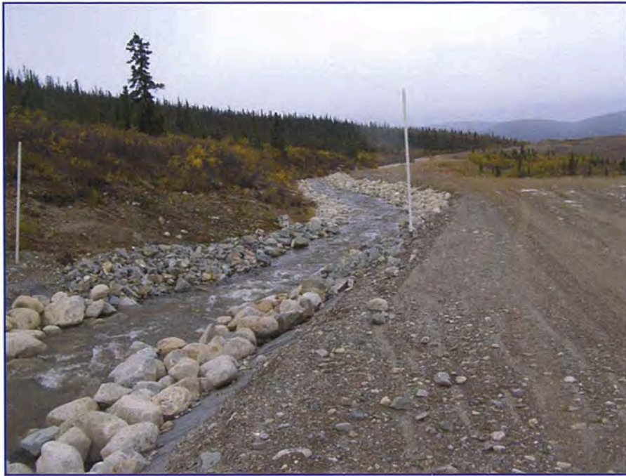
September: shows a view of Faro Creek Diversion Channel looking downstream.
