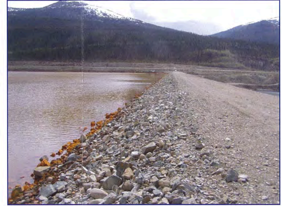
May: a view looking south along the upstream face. Note that the pond level appears to be close to the high water mark.
