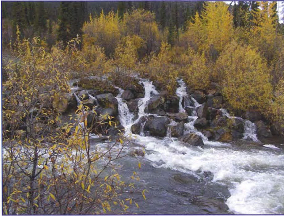
September: view of the left bank riprap in lower weir section, this is where Severin Creek enters the Diversion Canal.
