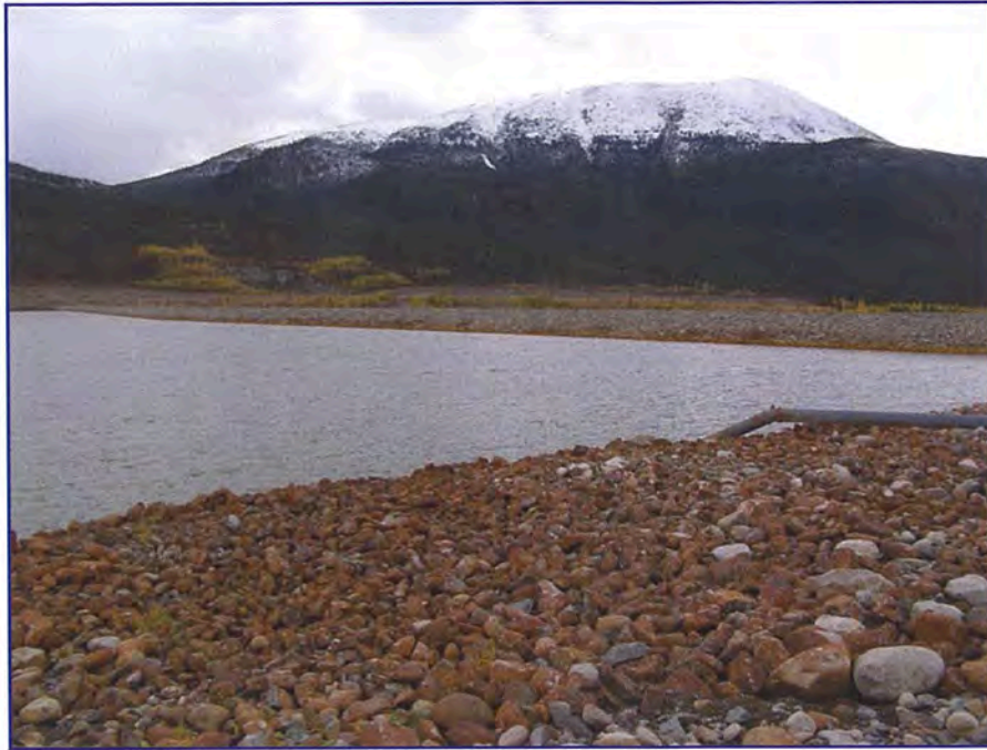
September: shows a view of the upstream face of the dam.
