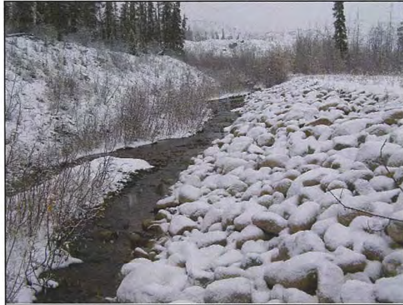
September: shows the start of the north Valley Interceptor Ditch just uphill from the guard house gate. This is the area the dike was repaired before and the riprap is obvious on the right hand side of the photo. After inspection of this section, it appears that the channel is flowing quite well with no signs of erosion or blockages.
