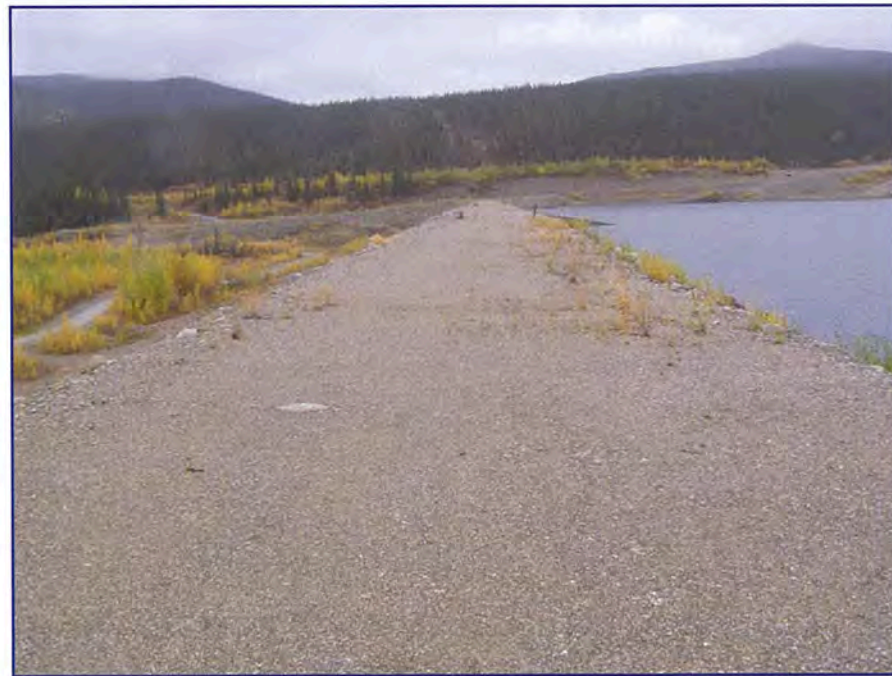
September: shows the crest of the dam, note that vegetation was removed in 2007.
