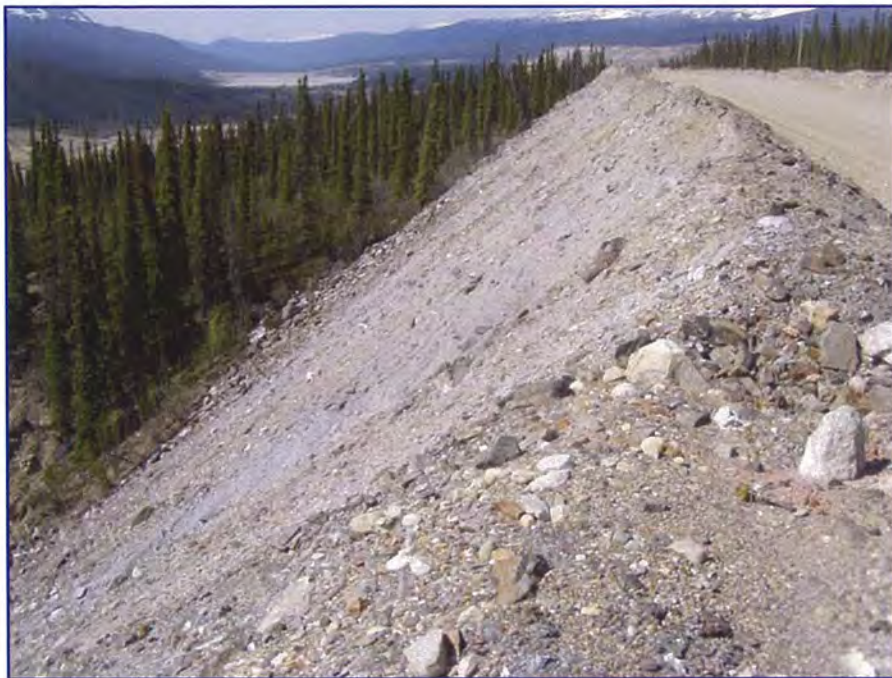
June: shows the overall slope of the downstream side of the rock drain
