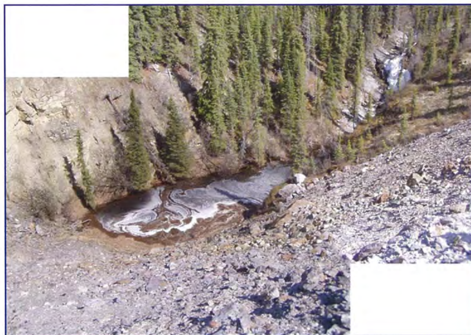
June: a view looking down the upstream face of the rock drain at the upstream pond.
