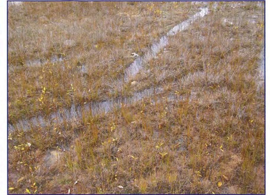
September: shows seepage water exiting the downstream toe about 12-14 m downstream of the seepage collection ditch. This area is slightly lower in elevation than the main channel containing seepage water but likely part of the same seepage path. Site staff to watch this area carefully in the winter.
