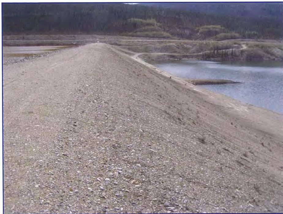
May: showing a view looking south along the downstream dam face.
