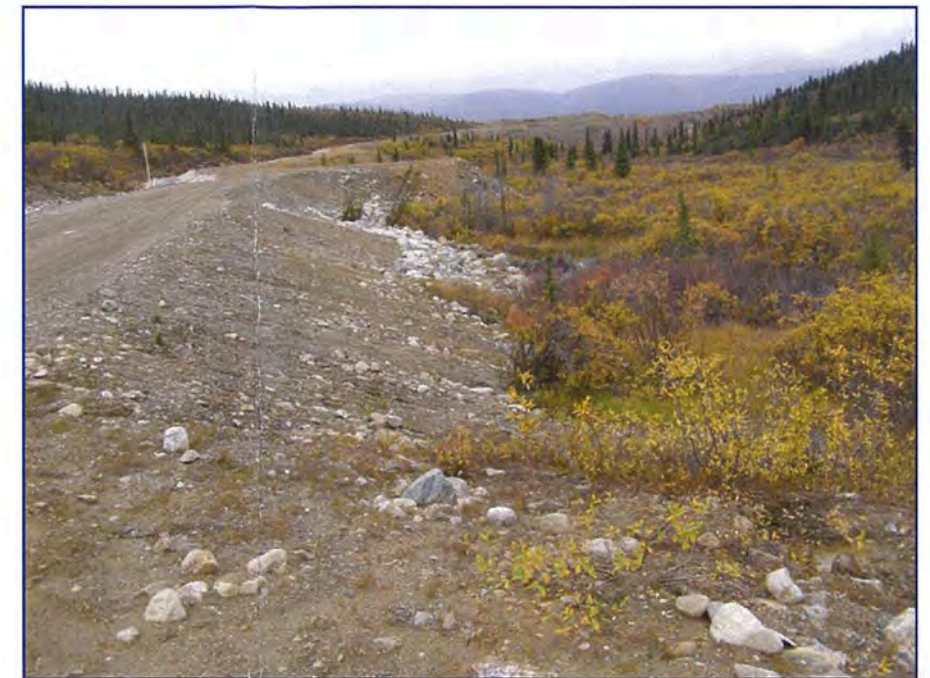
September: shows the toe of the road in the repair area. Note the ponded water in the toe area.
