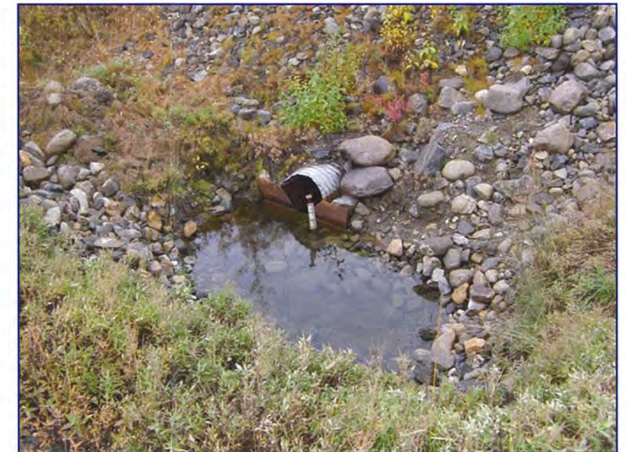
September: shows the seepage discharge weir and staff gauge. Staff gauge read 0.072 m.
