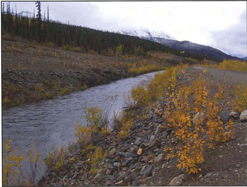
September: shows the water flowing in the channel section, looking in the downstream direction from downstream of the Diversion Dam.
